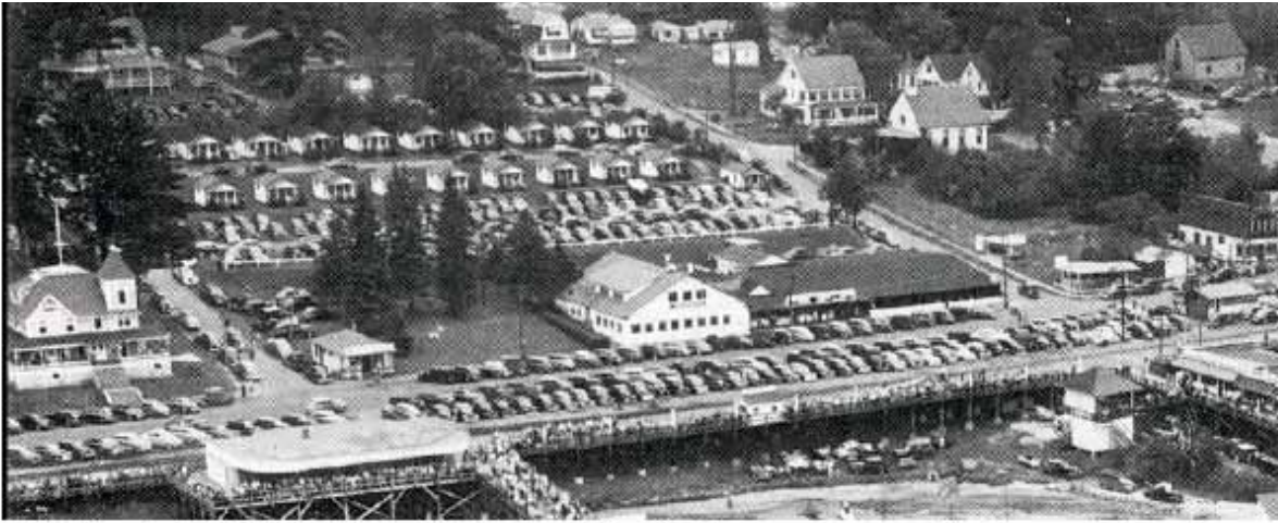
Weirs Beach Waterfront – As this image illustrates, parking challenges are not new to the area. Source: www.weirsbeach.com
