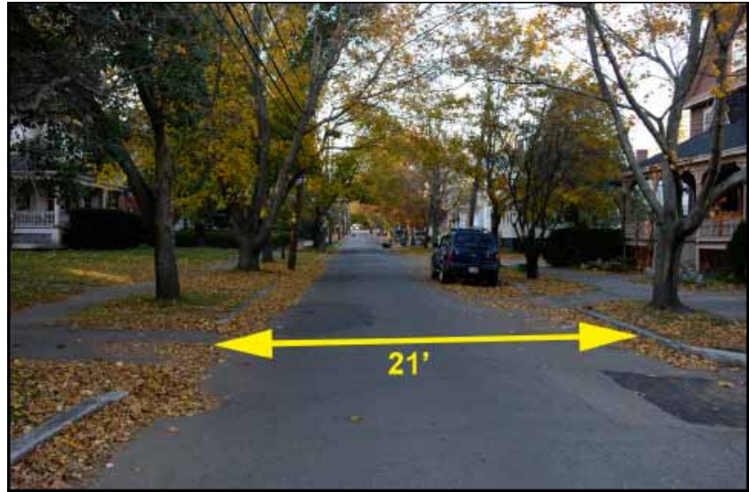
This cross-section of a yield street showing how a narrower street can accommodate two-way traffic and parking on one side. Since the traffic demand is lower, cars yield to one another when passing the parked vehicle, inducing traffic calming, and smaller, cozier neighborhoods.
