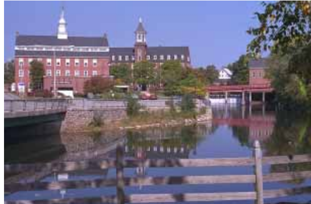
A view of the restored Belknap Mill building.
