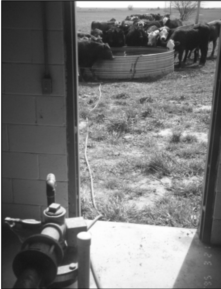
When livestock are allowed to feed near a drinking water well, the source water can possibly become contaminated with pathogens.
