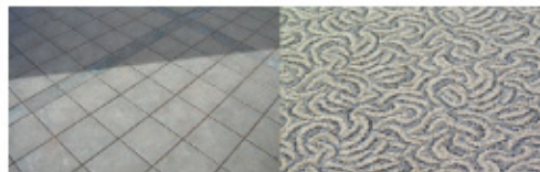
Low volatile organic compound paint, adhesives, glues, carpet, and floor tiles were used to finish the building. Absorbent materials such as carpet, ceiling tile, and furniture were installed after chemical odors dissipated.
