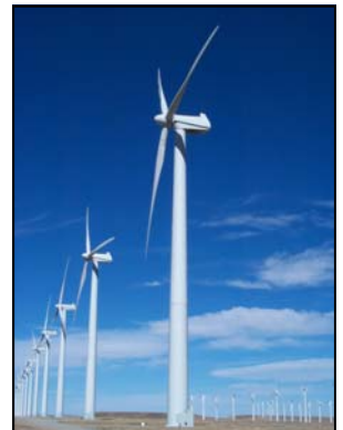
Foot Creek Wind Power Project, Arlington, WY
