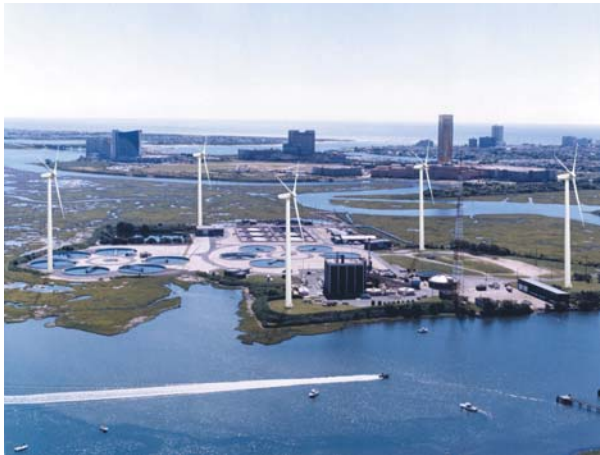
Figure 4. ACUA Wastewater Treatment Plant wind farm in Atlantic City, New Jersey.
