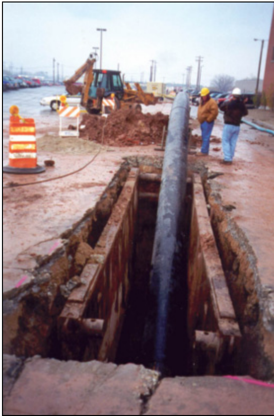
Courtesy of Earth Tool Company, LLC
