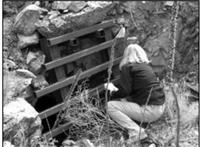
Other adits are fitted with “bat gates” to maintain the bat habitat but make it safe for the curious explorer. Here Eve Byron, a reporter with the Helena Independent Record, takes a closer look at a bat gate installed in the Scratchgravel Hills north of Helena. Photo by Marilyn Krause
