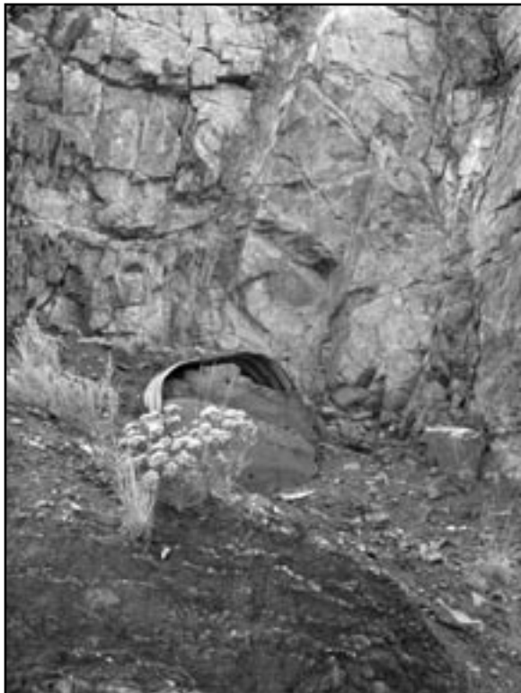
For safety reasons, some adits are closed completely with expandable insulation material. Photo by Marilyn Krause
