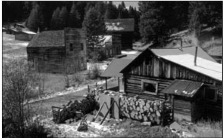
The historic Dahl Cabin (on the right) in Garnet is available for rent from December to April.
