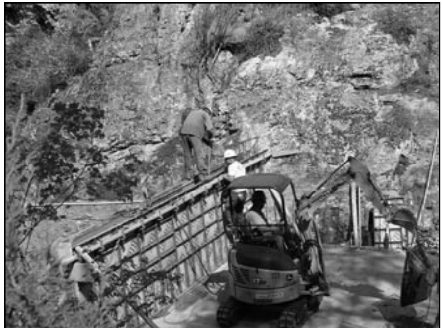
Construction in progress on the Crooked Creek fish barrier.
