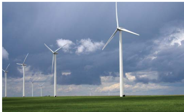
Wind farms like this one near Lamar, Colorado, provide electricity without producing carbon dioxide emissions. NSF researchers are exploring new ways to incorporate alternative energy sources, such as wind farms, into the national power grid. Credit: Bob Henson
