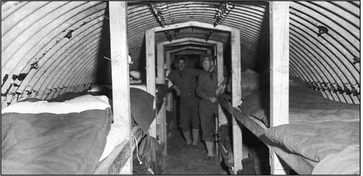
Once on high alert, Fort Cronkhite soldiers manned their guns around the clock. This photo shows the men's sleeping arrangements on Wolf Ridge, in a temporary corrugated metal shed, similar to a Quonset hut, built into the side of the hill. Photo 1942.
