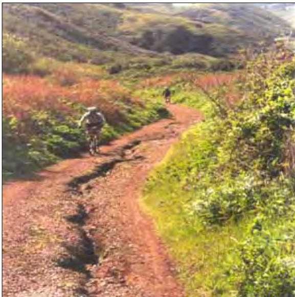
Photo 1.13 Severe trail erosion on Julian Road.
