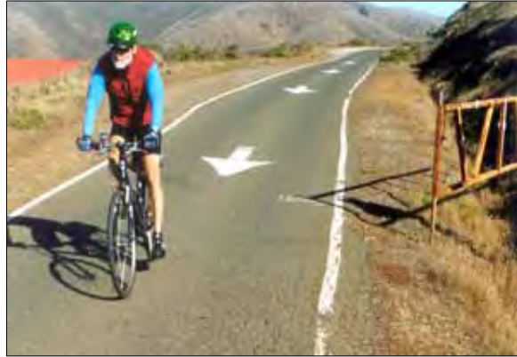
Photo 1.7 Bicycling on the narrow Conzelman Road (west of Hawk Hill), with deteriorating pavement.
