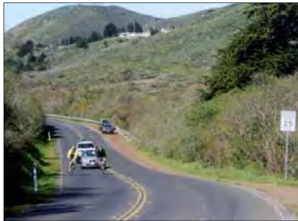
Photo 1.8. Lack of bicycle facilities on Bunker Road.
