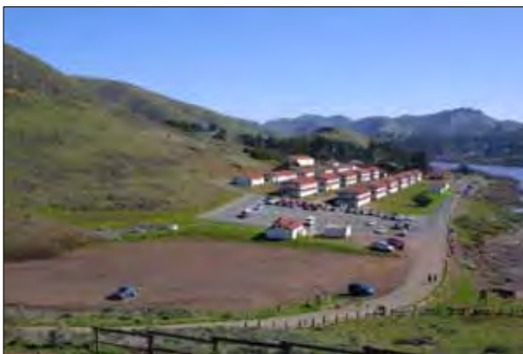
Photo 3.7. Fort Cronkhite from the Coastal Trail.
