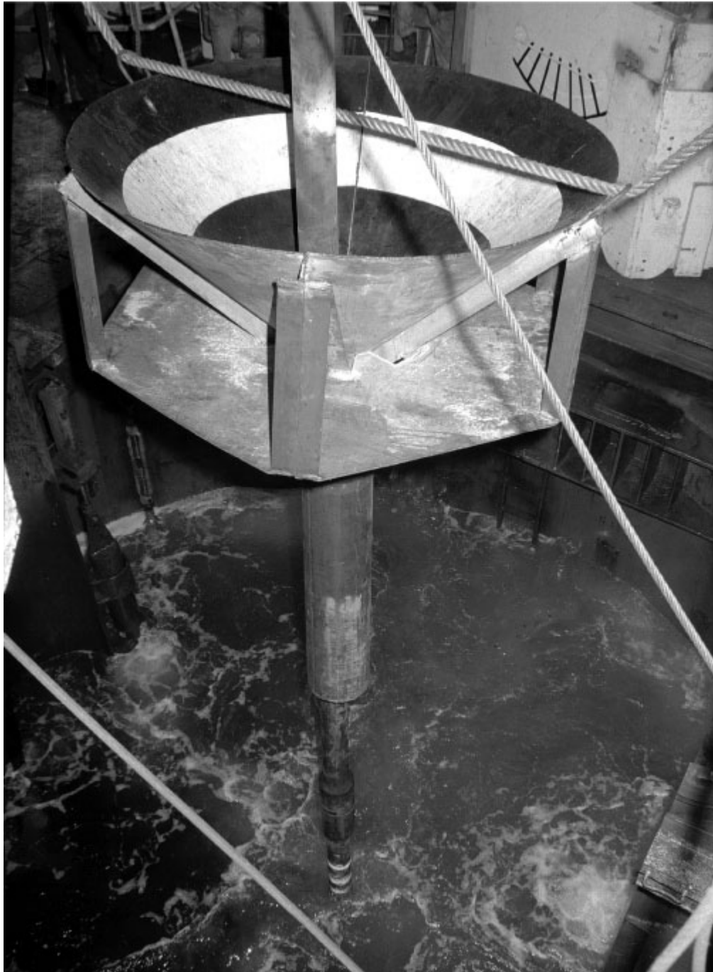
Figure 2. FFF with a 9 ft casing stub installed over the drill string and ready to drop in the moonpool.
