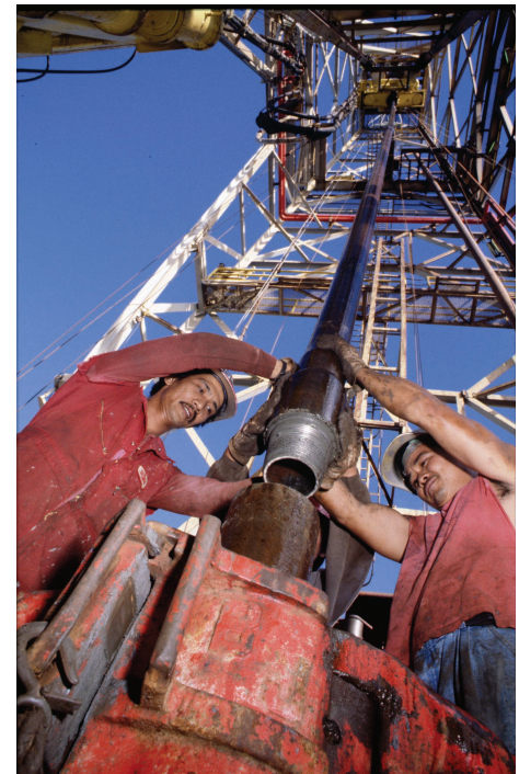
Figure 4. Making a drill pipe connection on the rig floor. The elevator (red clamp at the bottom of the picture) supports the box [or upper] end of the drill pipe and holds the weight of the entire drill string during a connection.
