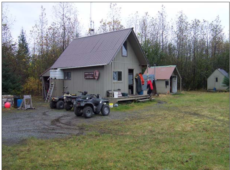
Figure 9. Existing Ranger Station. The facilities support NPS operations in Dry Bay.
