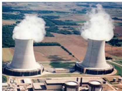
Thermoelectric cooling towers
