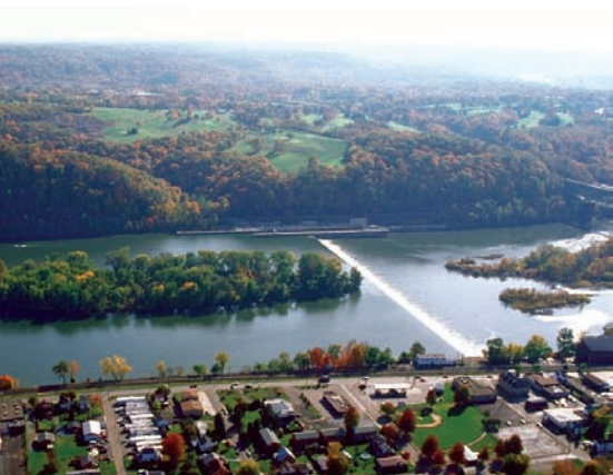
Navigation lock and dam on Allegheny River, Pennsylvania
