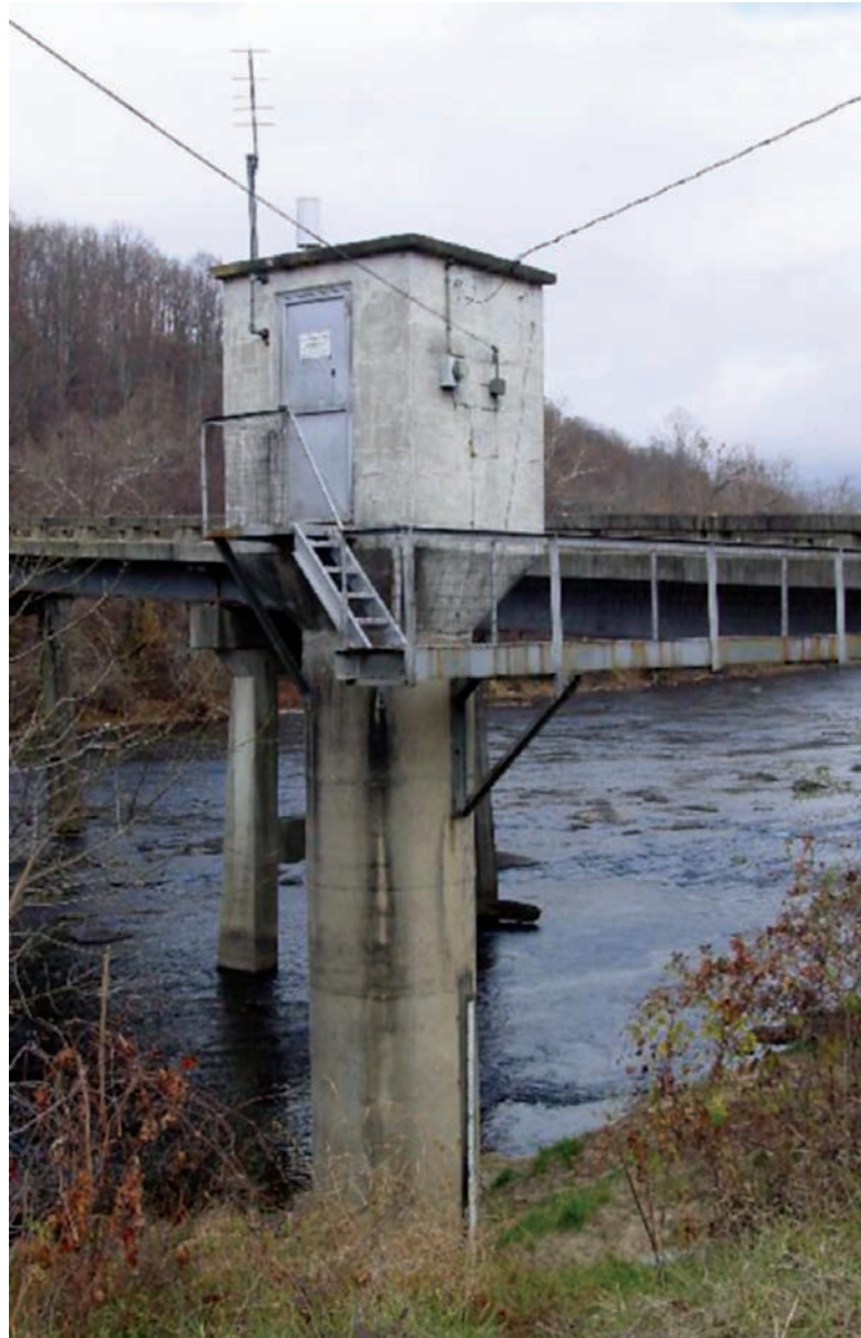
French Broad River at Asheville, North Carolina. Long-term hydrologic records are used to establish flow status and trends. The USGS has measured streamflow at this site from 1895 to present; current real-time measurements are made in cooperation with the Tennessee Valley Authority.
