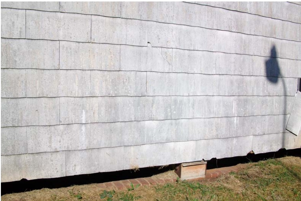
Photograph No. 2: Possible asbestos containing material (ACM) shingles on exterior of Warehouse No. 1.
