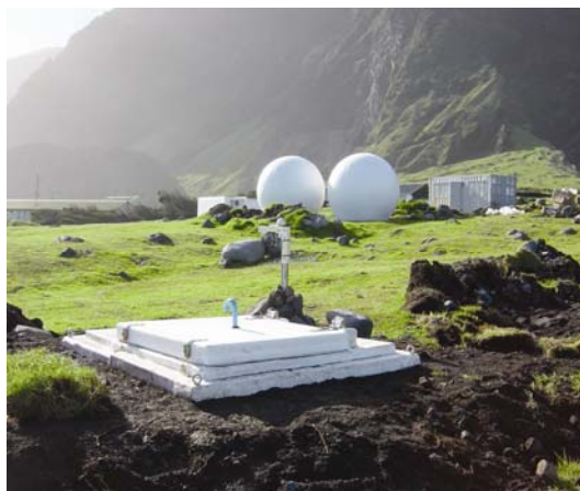
This is an image of the entrance to the Global Seismic Network's seismic vault on Tristan da Cunha in the South Atlantic. This station is part of a collaboration with the Comprehensive Test Ban Treaty Organization International Monitoring System and Geoscope. Credit: Ted Kromer.
