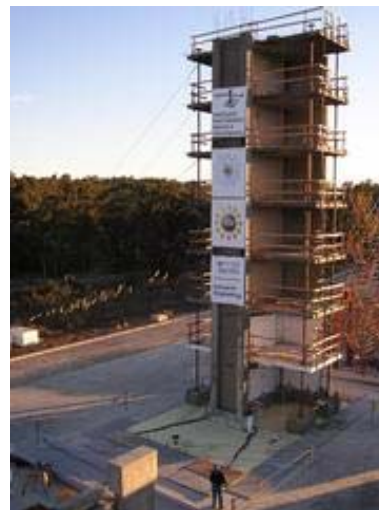
The seven-story, 275-ton reinforced concrete structure tested on the University of California, San Diego NEES shake table demonstrated a less costly seismic design method for residential structures in southern California. Credit: Professor Jose estrepo, Department of Structural Engineering, UCSD
