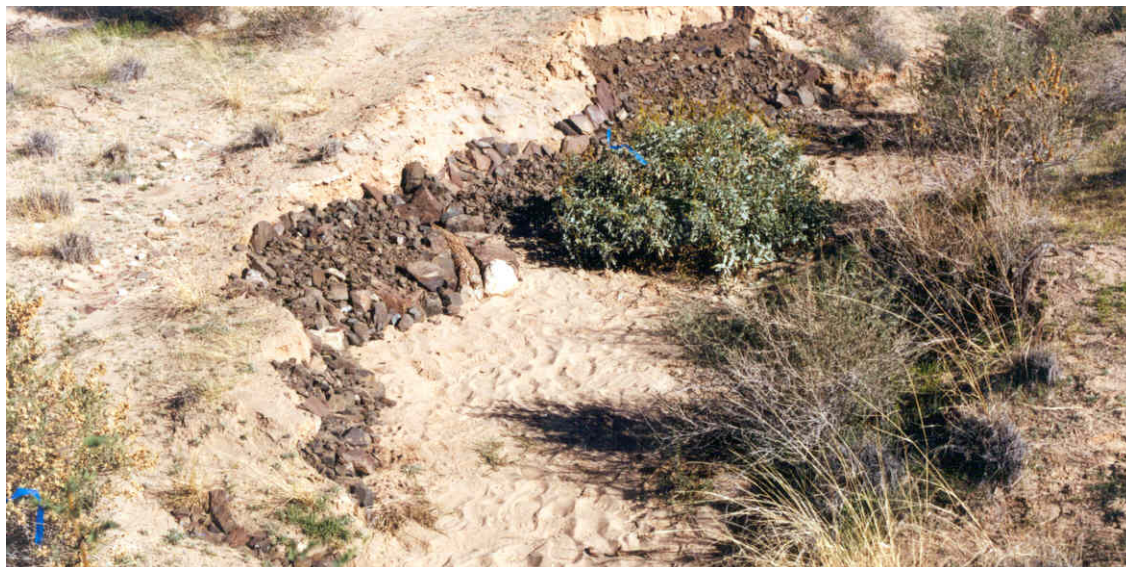
Figure 7. A checkdam protecting a cutbank adjacent to an archaeological feature.
