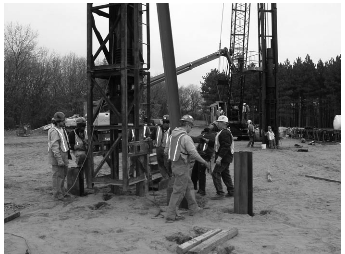
Piledriver operators use large machines to hammer piles into the ground.
