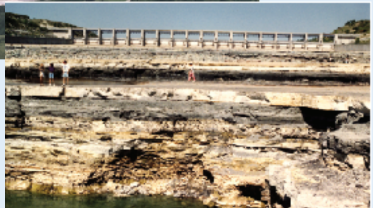
(A) Controlled flow over the emergency spillway at Tuttle Creek Lake, north of Manhattan, July 1993 (photograph courtesy of Paul Maginness, Photographic Services, Kansas State University, Manhattan, Kansas) and (B) reservoir releases cut 20-foot-deep canyon in solid rock downstream from Tuttle Creek Lake, July 1993 (photograph by Charles A. Perry, USGS)
