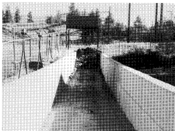
Figure 6.—Concrete test stope and festoon system.
