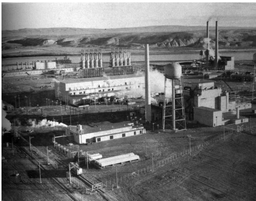
Figure 1-4. 100-F Area in 1944. Initially, three plutonium-producing reactors were built, about six miles apart, on the south bank of the Columbia River. At each site, in addition to the reactor buildings, there were electrical substations, pump stations, water treatment plants, retention basins, and waste processing plants. Department of Energy photo from Fermi and Samra (1995) .
