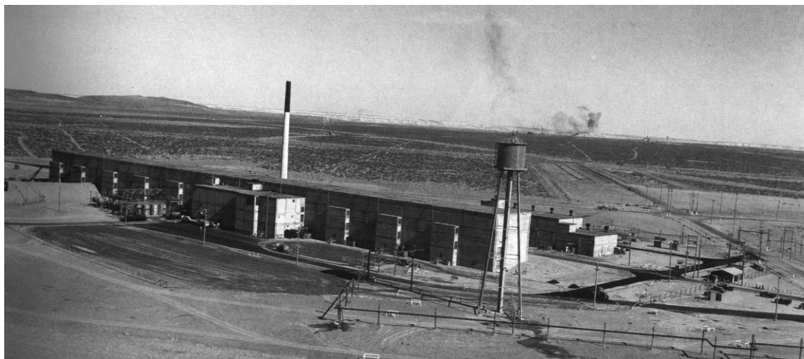
Figure 1-5. Fuel processing (T) Plant in 200–West Area in 1944. Rail cars brought the irradiated uranium slugs from the production reactors in 100 Areas to the separation areas in large vats of water. Here, they were stored in pools of water to allow some of the intense, short-lived radioactivity of the fission products to decay before processing. Department of Energy photo from Fermi and Samra (1995).
