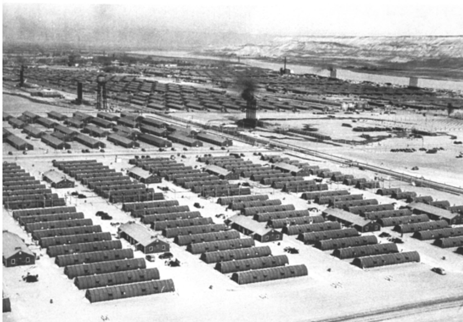
Figure 3-3. View of Hanford construction camp, with barrack hutments in foreground. “Hutments” was a term for the fabricated temporary buildings, which later were referred to as “Quonset huts” because the first of that type in this country had been built at Quonset, Rhode Island. The camp housed some 40,000 workers. The trailer camp was home to another 12,000 residents, including dependents. Hanford Camp was built in 1943 and abandoned in early 1945 when the construction period ended ( Sanger 1995).
