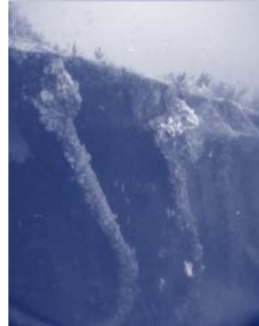
Bent and bowed deck support stanchions and the angled ends of "floor beams" along the port boiler.
