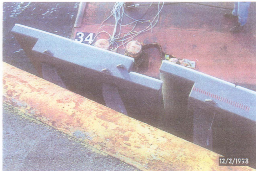
Figure F-2-2 Typical deflections of fender system during impact (top view)
