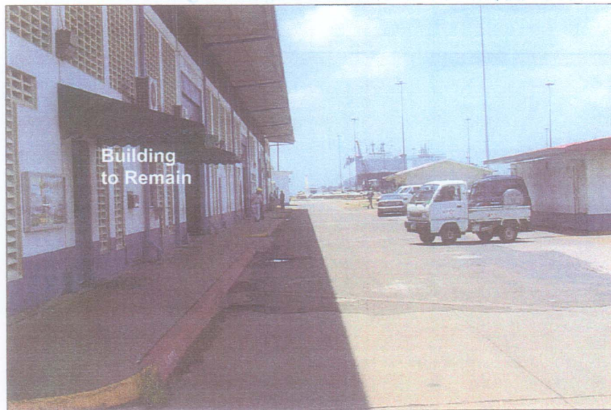
Figure D-1-4 Southern End Of Access Road, Which Extends Along Gatun East Wall
