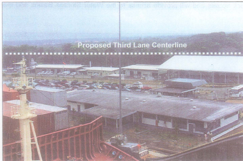
Figure D-1-6 Buildings Along Esplanade
