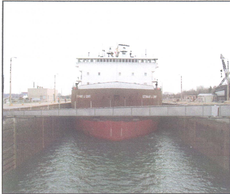
Figure B-2-2 Articulated Fender Boom in Front of Miter Gates
