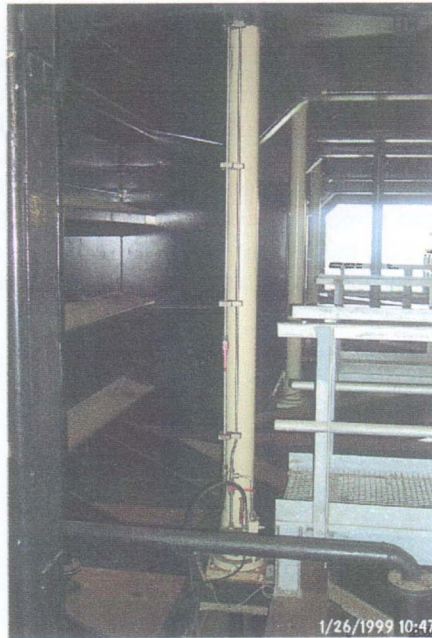
Figure B-2-8 Gate Mounted Filling/Emptying Valve Cylinders
