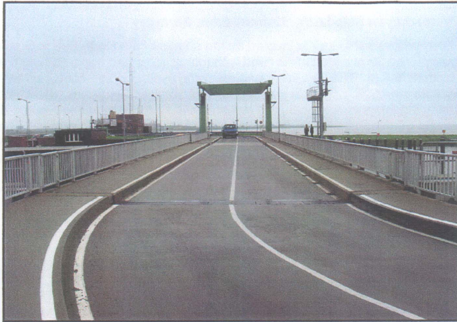
Figure B-2-4 View Looking Across Upstream Gates. Note Moveable Curved Roadway Section (See Figure B-2-5)
