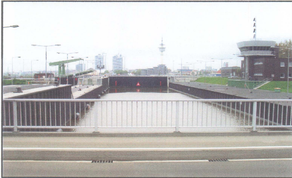
Figure B-2-3 Bremerhaven Ship Lock, Germany
