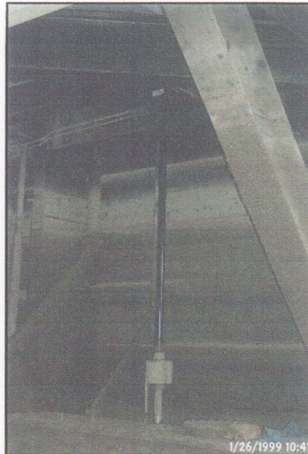
Figure B-2-9 Typical Bonnet and Cylinder Rod for Filling And Emptying Valves
