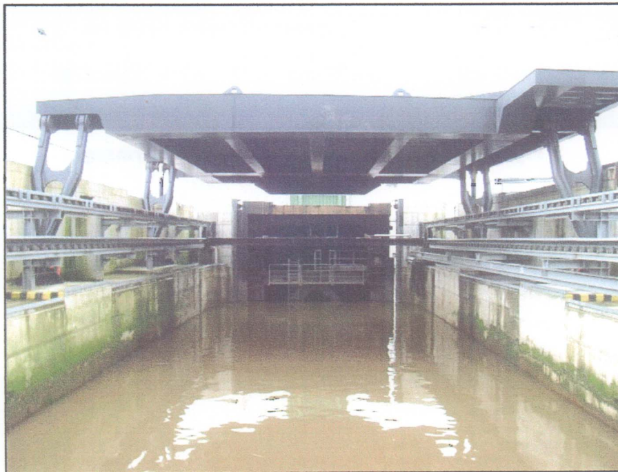
Figure B-2-5 Rolling Gate In Closed Position With Roadway Raised
