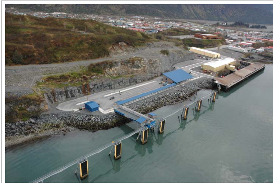
Forms An (ferry terminal), Asj (seawall, jetty), Ap (port facility), BC Class 32 Ferry terminal, Valdez (Unit 02/03/6241) PWS07_MM_07432.jpg
