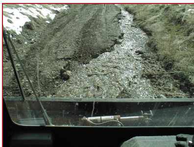
Pictures taken from the Snow Cat before the Road was improved. Water was gushing down and eroding the road in many areas making a harrowing trip to the RADAR site in the Snow Cat. Photo Courtesy Herb Loell
