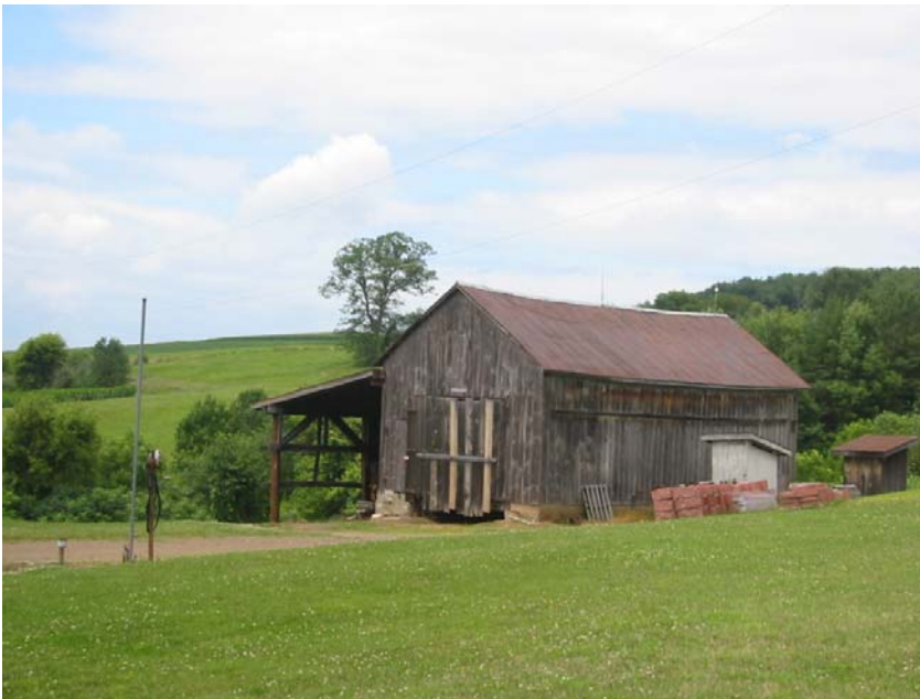
037-LO-002. Machine shed, Locust Township, Columbia County.
