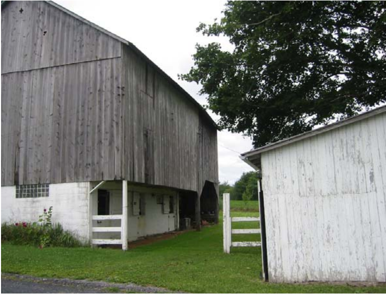
037-LO-001-03 N. Barn, looking SW, Locust Township, Columbia County. Note the machinery bay.
