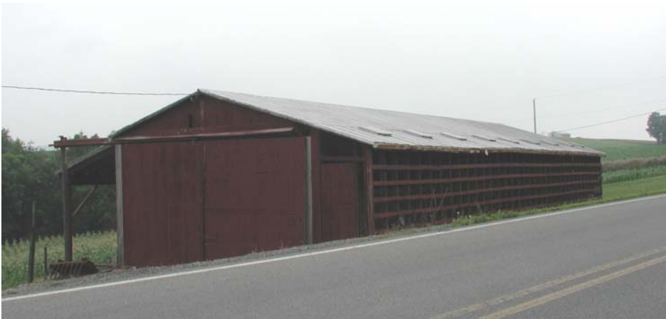
Machine shed- corn crib, Lower Mahanoy Township Northumberland County, site # 097-LM-004-14
