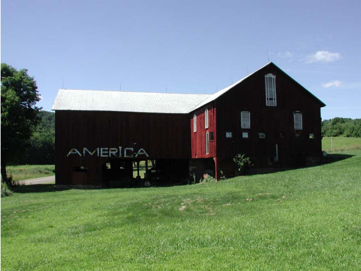
037-gr-004-15. Barn, America. This barn integrates hog house in the ell; poultry in the main wing; machinery bays; and stanchions. Greenwood Township, Columbia County
