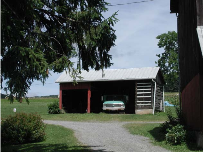
Machine shed and corncrib. Columbia County GR-002.
