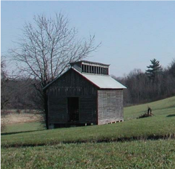
Union County corncrib with loading slots in clerestory arrangement.
