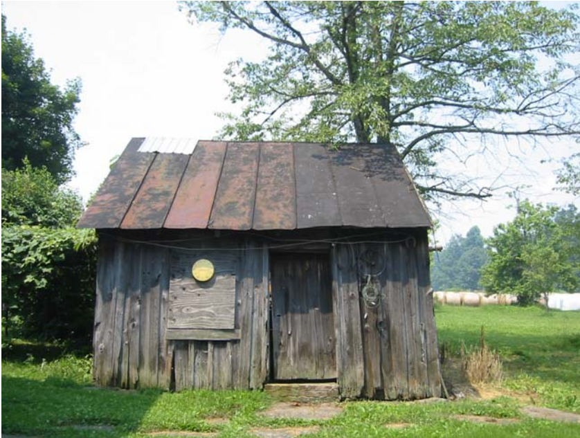
037-NC-001. North Center Township, Columbia County Butcher house. The roof patch could indicate a chimney.
