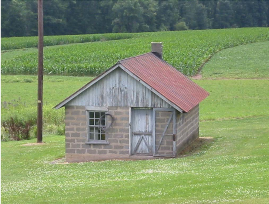
037-LO-002. Brooder House, Locust Township, Columbia County. This building has characteristic features: small size-- too small to be a summer kitchen--, windows, chimney, and siting close to the house.
