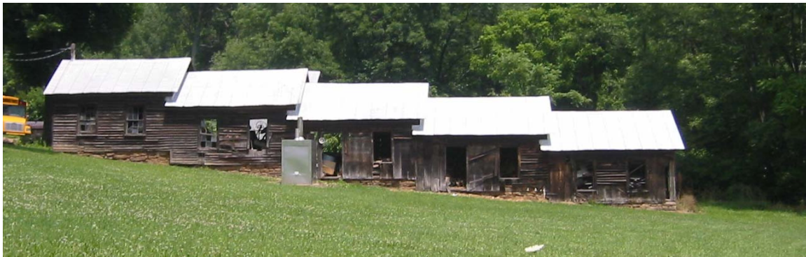
037-NC-001. Not typical, but notable. Poultry housing, North Center Township, Columbia County. This may have been a turkey house, note the image below.
