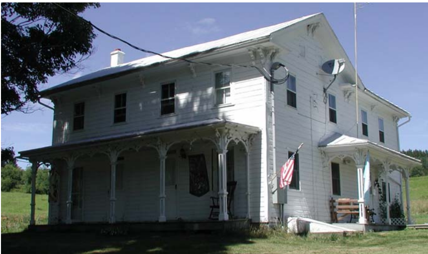
Columbia County, GR-005. A four-over-four with (in effect) not just two but four doors, if you consider the French doors flanking the two central doors. The owner dates it to the 1850s, which is probably close though the trim and 2/2 windows could place it a bit later. This house looks like it is two rooms deep but in fact the main section is only one room deep.
