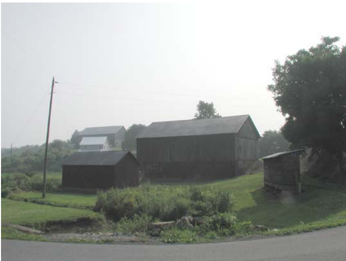
097-LM-006-01 91. Small cut road enhanced. Pennsylvania Barn, Lower Mahanoy Township, Northumberland County.
