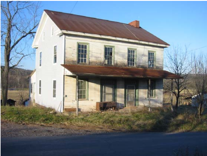
109-MI-001-11. House, looking N-NE. Snyder County. This four-over-four has two doors. Its six-over-six sash windows suggest a mid-19 th century date.
