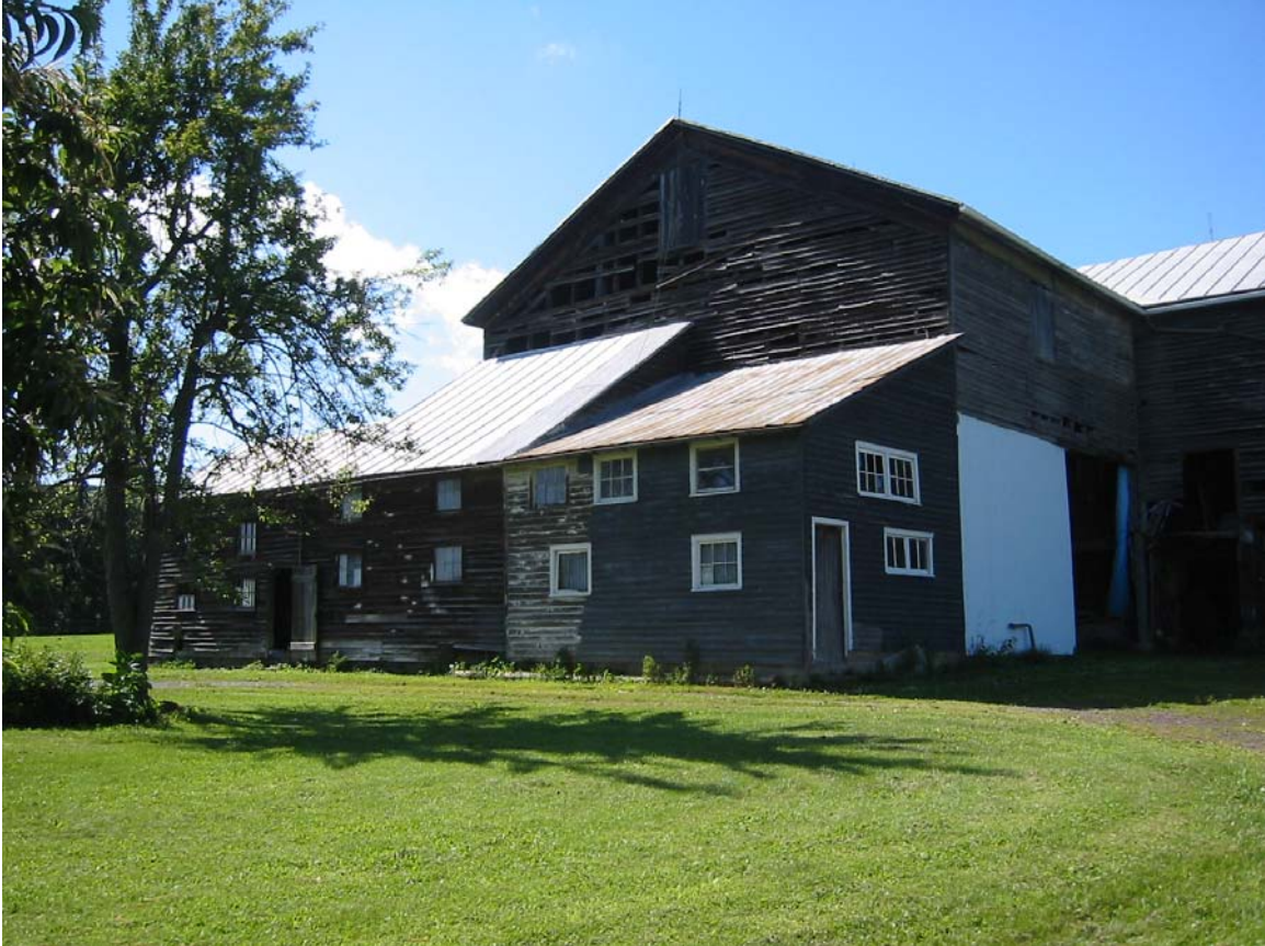
Site # 005 in Greenwood Township, Columbia County (above) contains two machinery bays; a straw shed; an outshed granary on the bank side; and two added shed-roof extension for poultry, added on to the straw shed.
