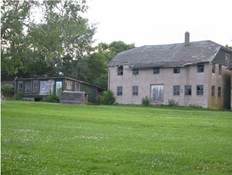
037-LO-006. Two poultry houses in Locust Township, Columbia County
