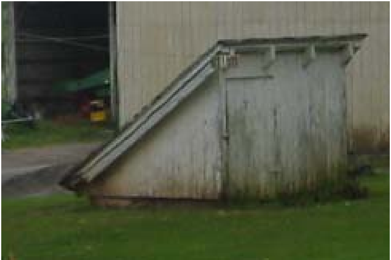
Possible root cellar, site # 081-MU-007, Muncy Township, Lycoming County
