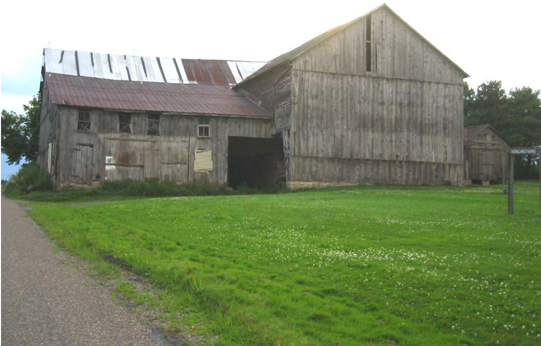
037-LO-006-06. Barn, Locust Township, Columbia County. The shed-roof extension suggests poultry housing and machinery storage, while the portion to the right seems to have originated as a Pennsylvania barn (the forebay is partially visible).
