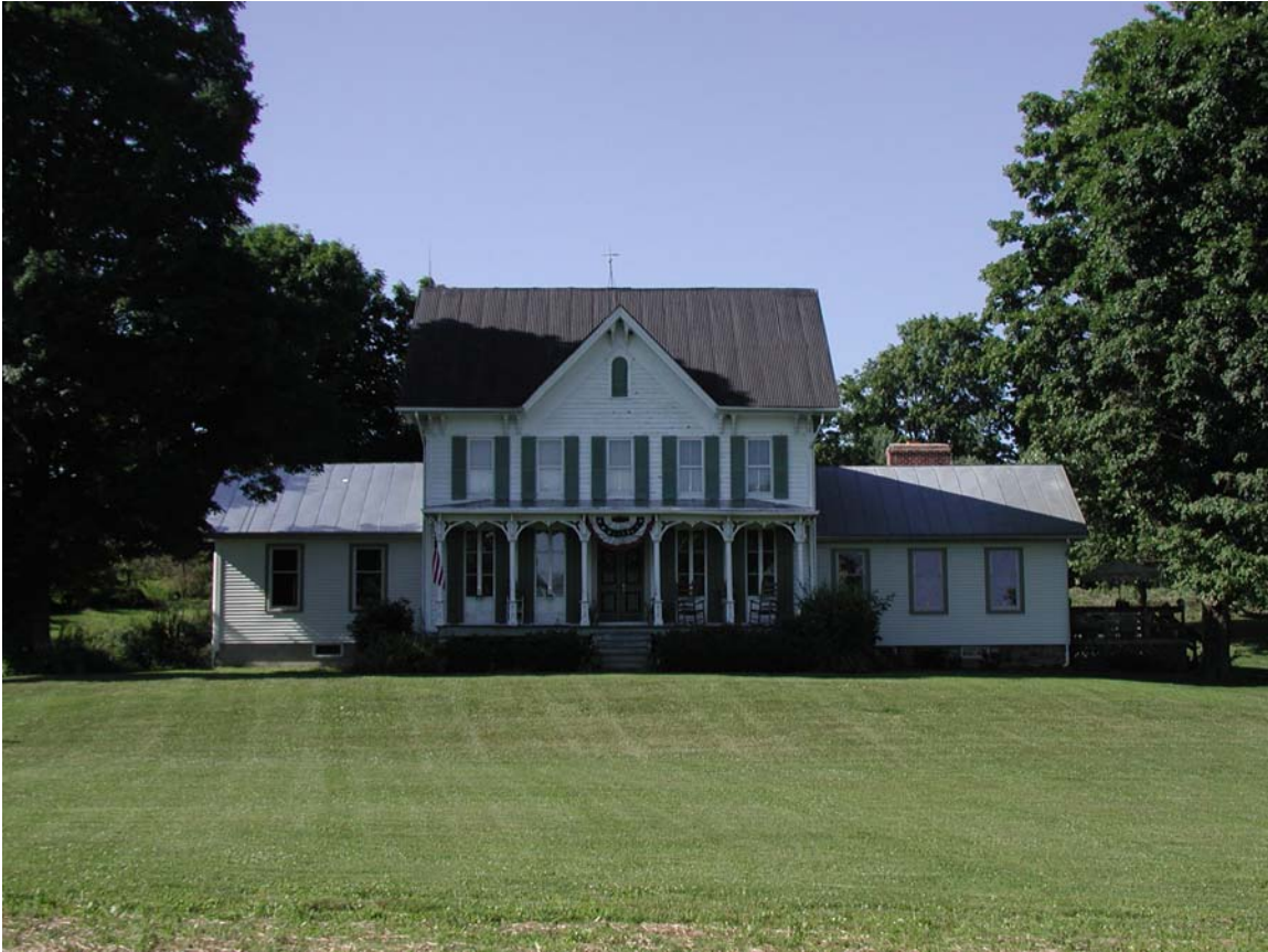
GR-006. House, Greenwood Township, Columbia County, c. 1867, features a by now standard look, updated with center gable, French doors, 2/2 windows, and bracketed porch and cornice.
