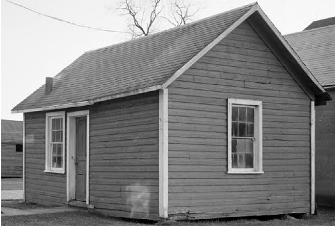
Summer kitchen, Probst farmstead, Clinton County, c 1916. HABS photo by Rob Tucher, 1991. Historic American Buildings Survey website, Survey number HABS PA-5523-B. Note door, windows, and chimney. Kitchen is located near main house. According to HABS (Historic American Buildings Survey) documentation, this kitchen was used for canning, storage, and other related activities. Its use declined after electrification in 1936.
