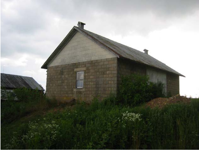
037-LO-004-14. Machine shed with root cellar below, looking SW. Locust Township, Columbia County. This machine shed was constructed of moulded concrete brick.
