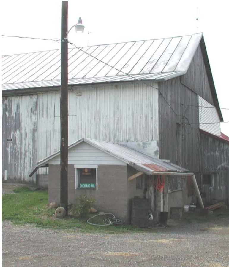
Greenwood Township, Columbia County. Concrete block milk house. Note the relationship to the barn.
