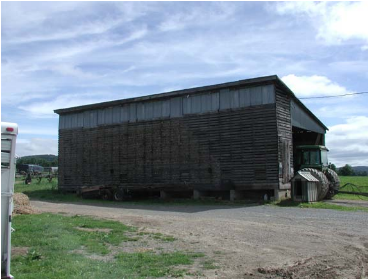
Columbia County, Greenwood Township # 001, corncrib
