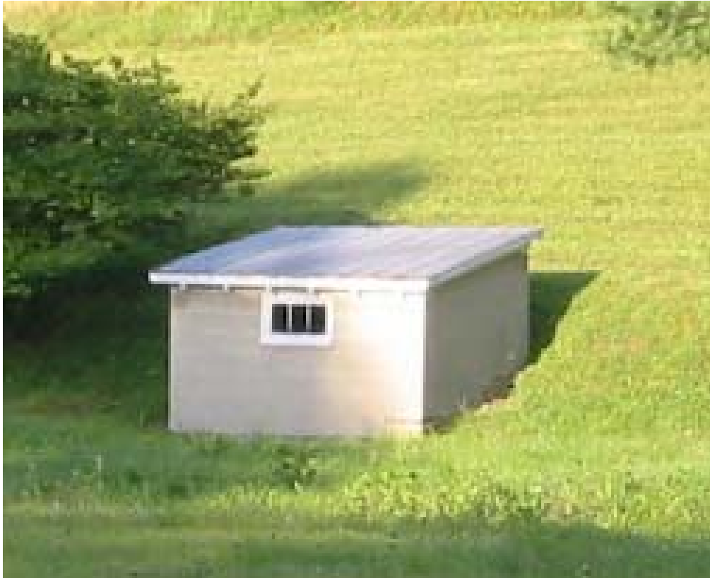
037-LO-005-06. Concrete block spring house. Locust Township, Columbia County.
