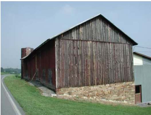
Pennsylvania Barn, Northumberland County, LM005. (left) This barn has one corner intact of log construction, and a datestone of 1845. The log end probably predates 1845.
