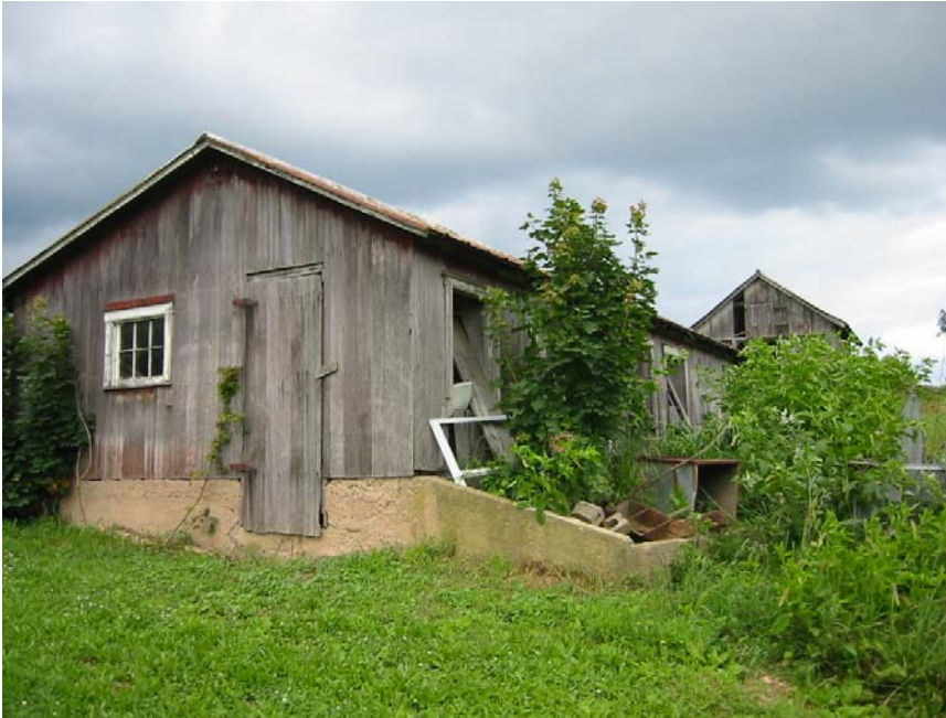
037-LO-004. Hog house, Locust Township, Columbia County. Concrete walls bound the run area.
