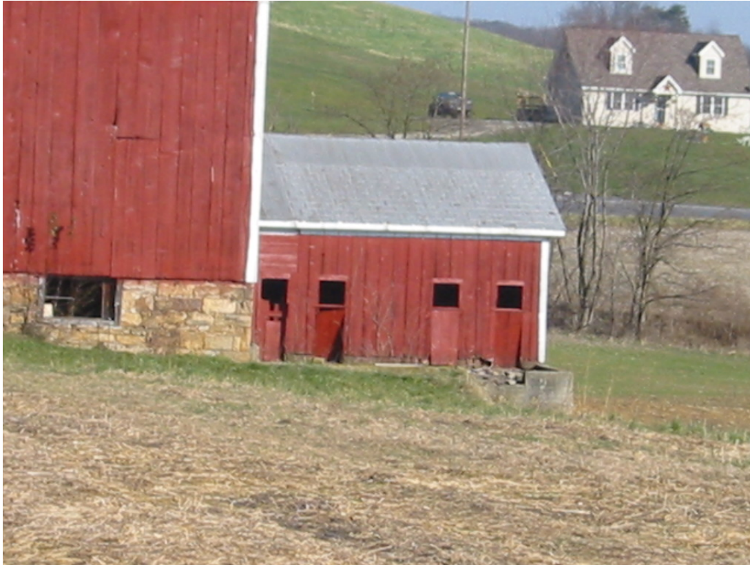
109-UN-001-16. Hog house. Union Township, Snyder County. This pen is in a common location, extending from the forebay of a Pennsylvania Barn.
