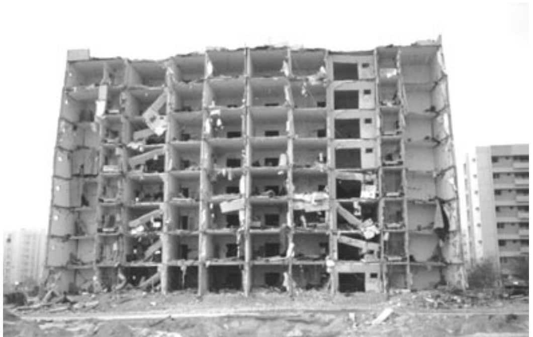
June 25, 1996—Dhahran, Saudi Arabia: Aftermath of the bombing of the al-Khobar military housing complex.
