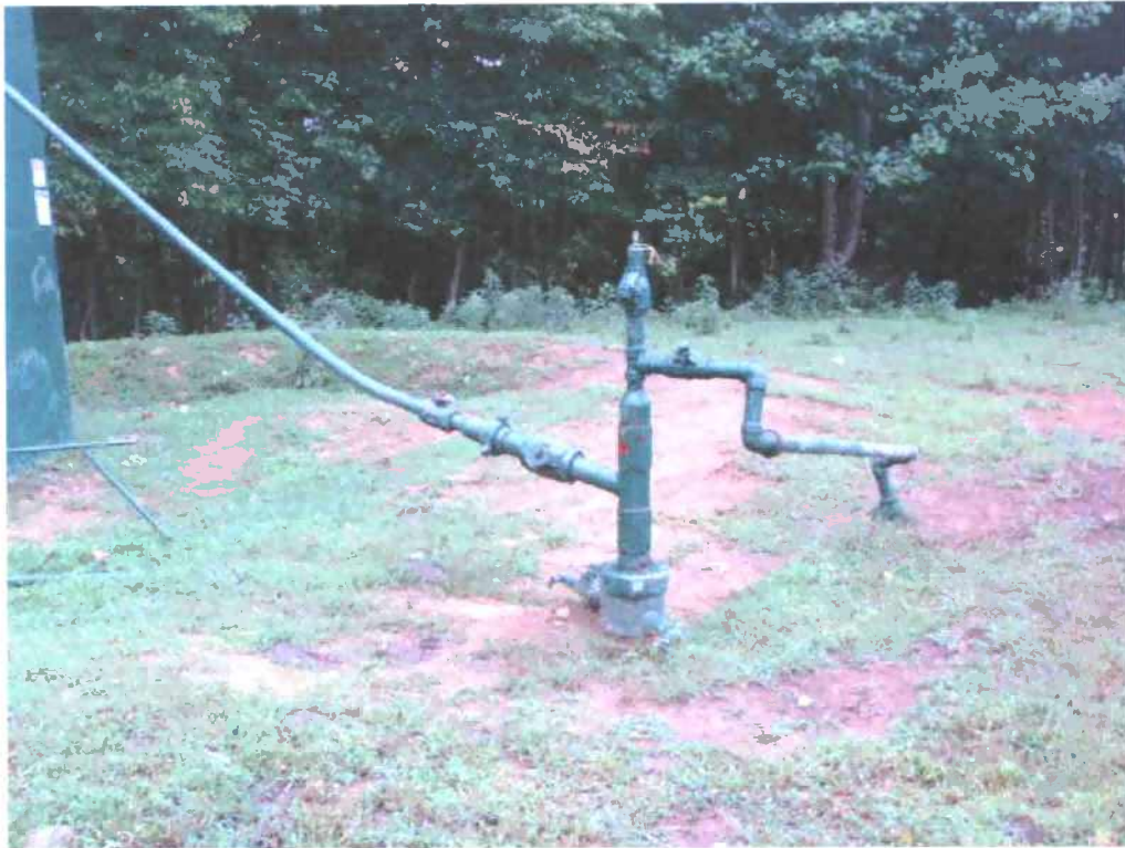
Figure 3. Keyspan well located 2,800 feet north-northwest of 6:26:35 a.m. Vaisala lightning strike location that shattered a large tree. Well is serviced by an approximate 3-inch diameter metal pipe that is buried until exposed at a monitoring station 300 feet to the northeast. No evidence of lightning damage was apparent to the metal, or the surrounding trees and ground.
