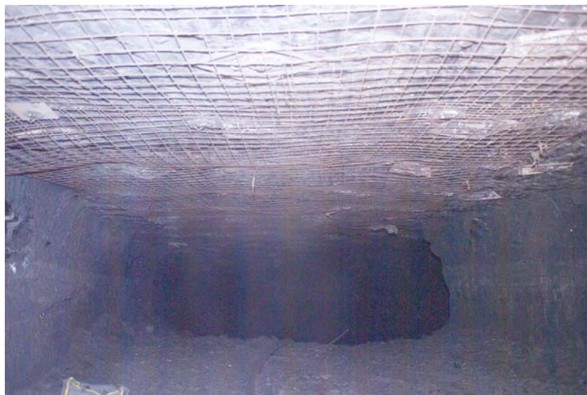
Figure 47 - Picture Taken Near Survey Station 4011
