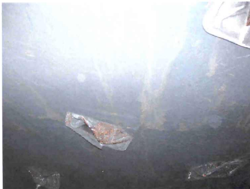
Figure 8. Photo of linear, wavy brown streaks in the terminated #8 Entry, viewed looking inby along #8 Entry. Streaks are actually the exposed bases of the brown shale that overlies the thin black carbonaceous shale bedding parting.
