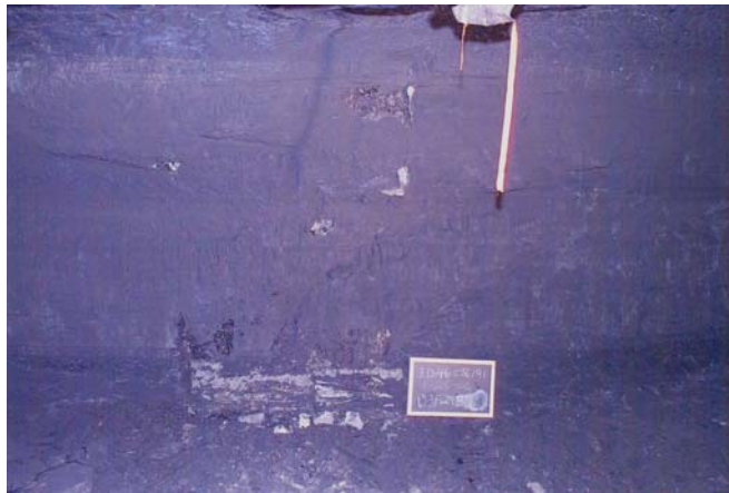
Figure 29 - Post-Explosion Location of Seal No. 10
