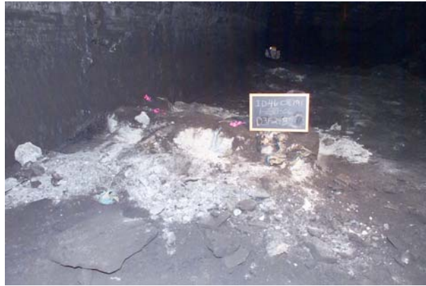
Figure 21 - Post-Explosion Location of Seal No. 2
