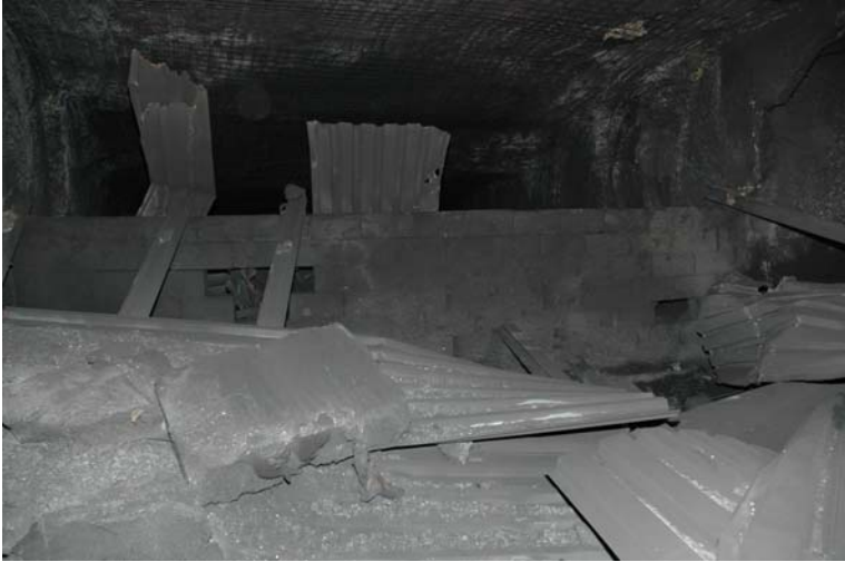
Figure 7 - Damaged Overcast at 58 Crosscut, No. 4 Belt
