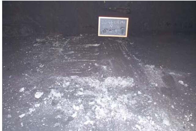
Figure 23 - Post-Explosion Location of Seal No. 4
