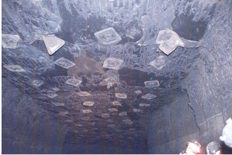
Figure 46 - Picture taken Near Survey Station 4010
