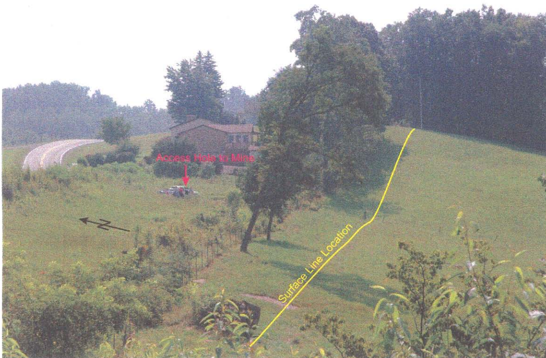
Figure 3. Photo of HRR survey line area. View is towards the east.
