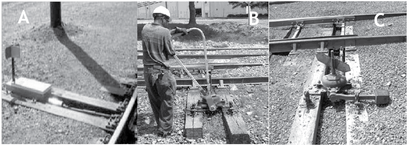
Figure 1. Switch designs: (a) old-style switch requiring awkward bending, (b) “bowtie” switch, (c) solar-powered (automated) switch.
