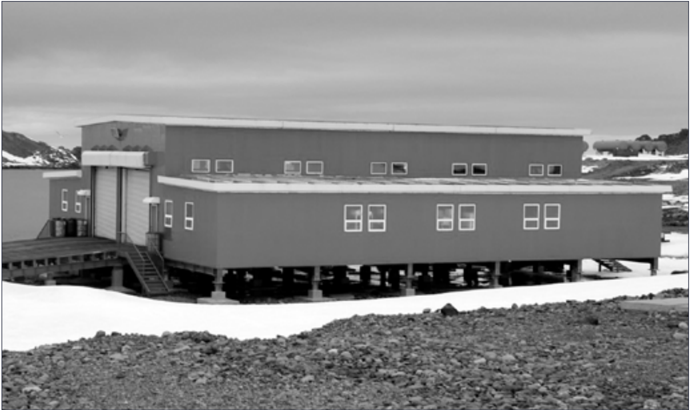
Great Wall Station, building and fuel tanks
