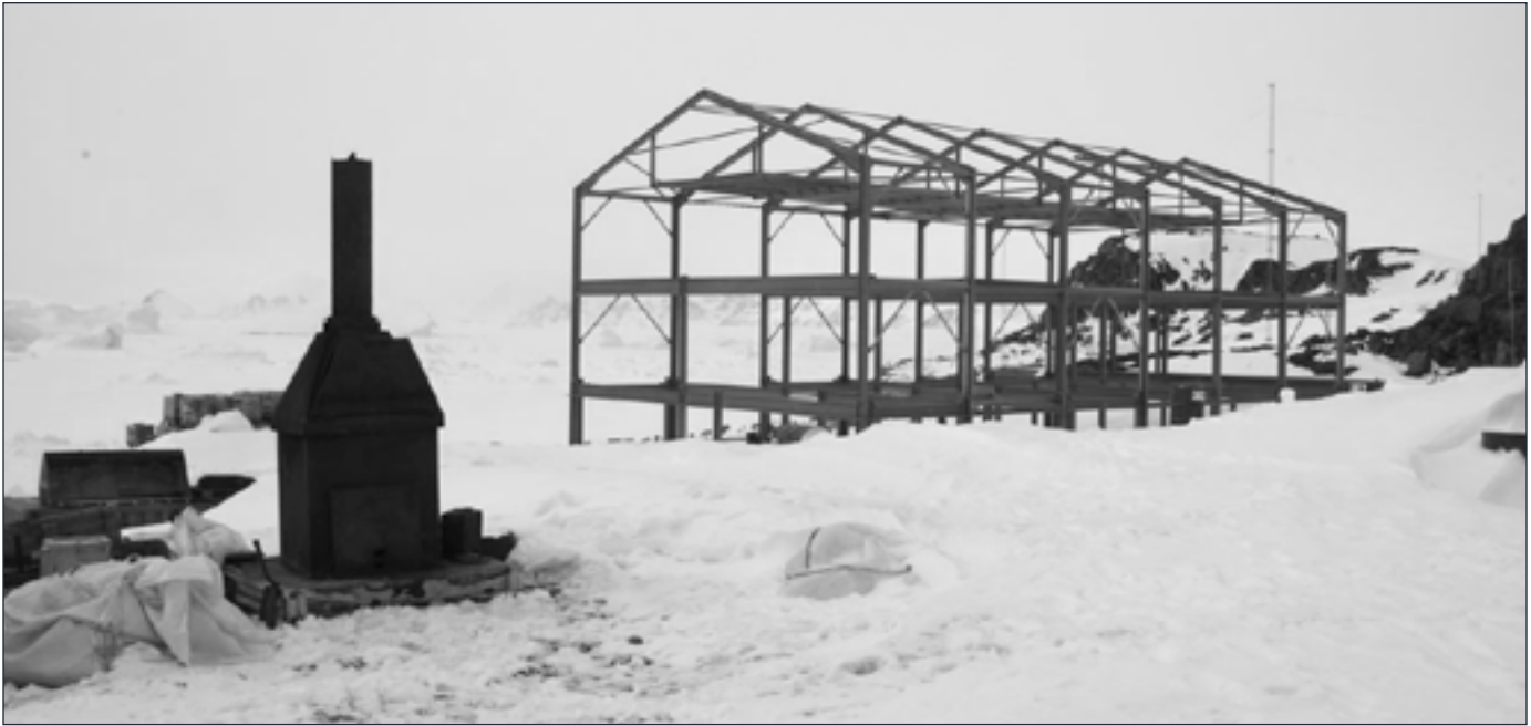
Rothera Station, construction of New Bransfield House and incinerator
