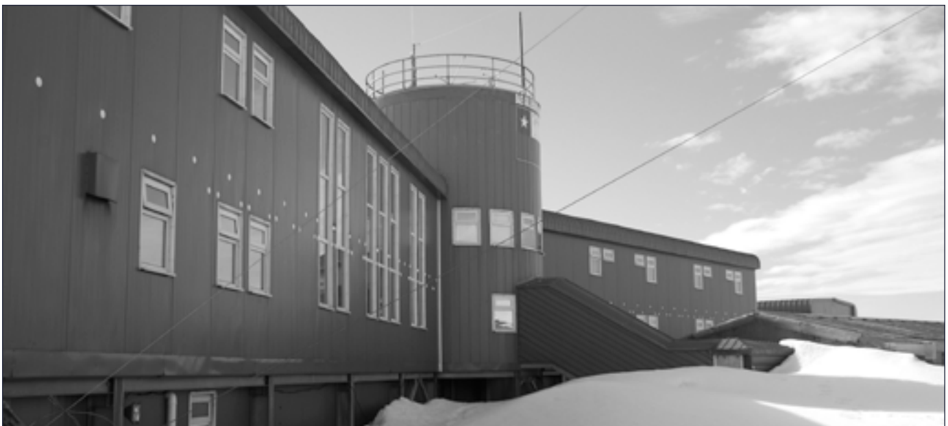
O'Higgins Chilean Station, new main building
