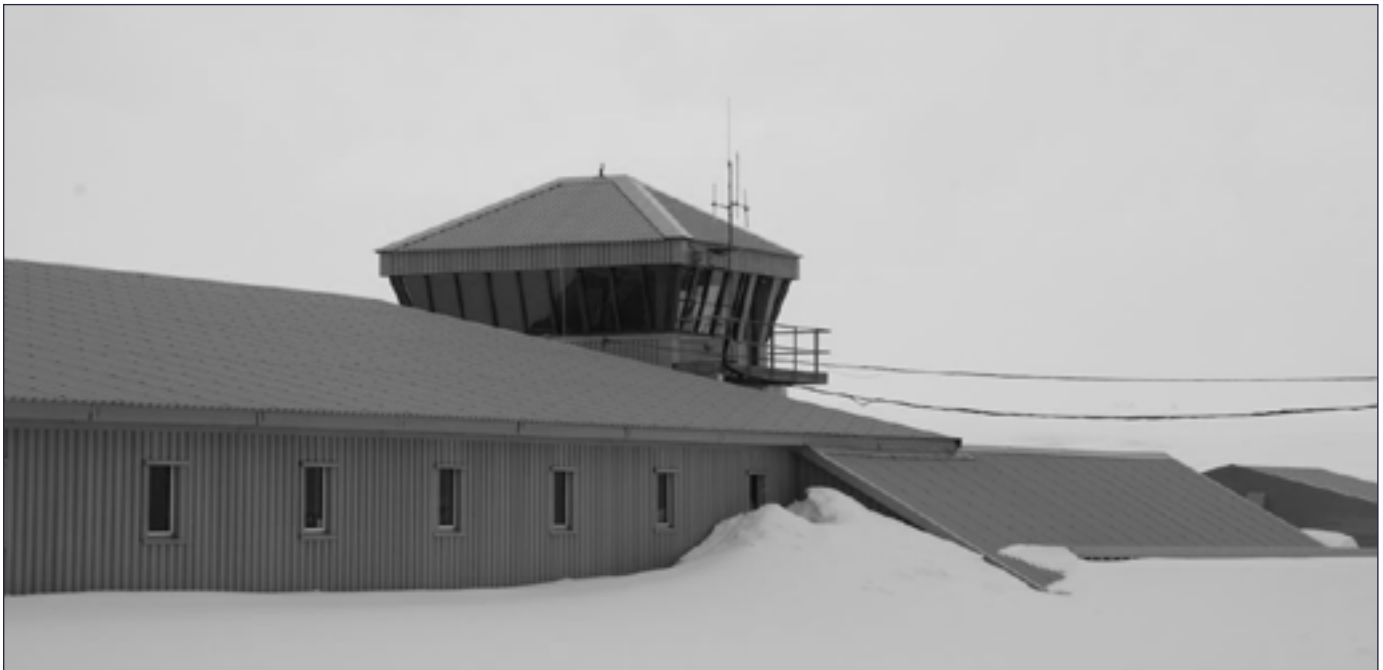
Rothera Station, Bransfield House
