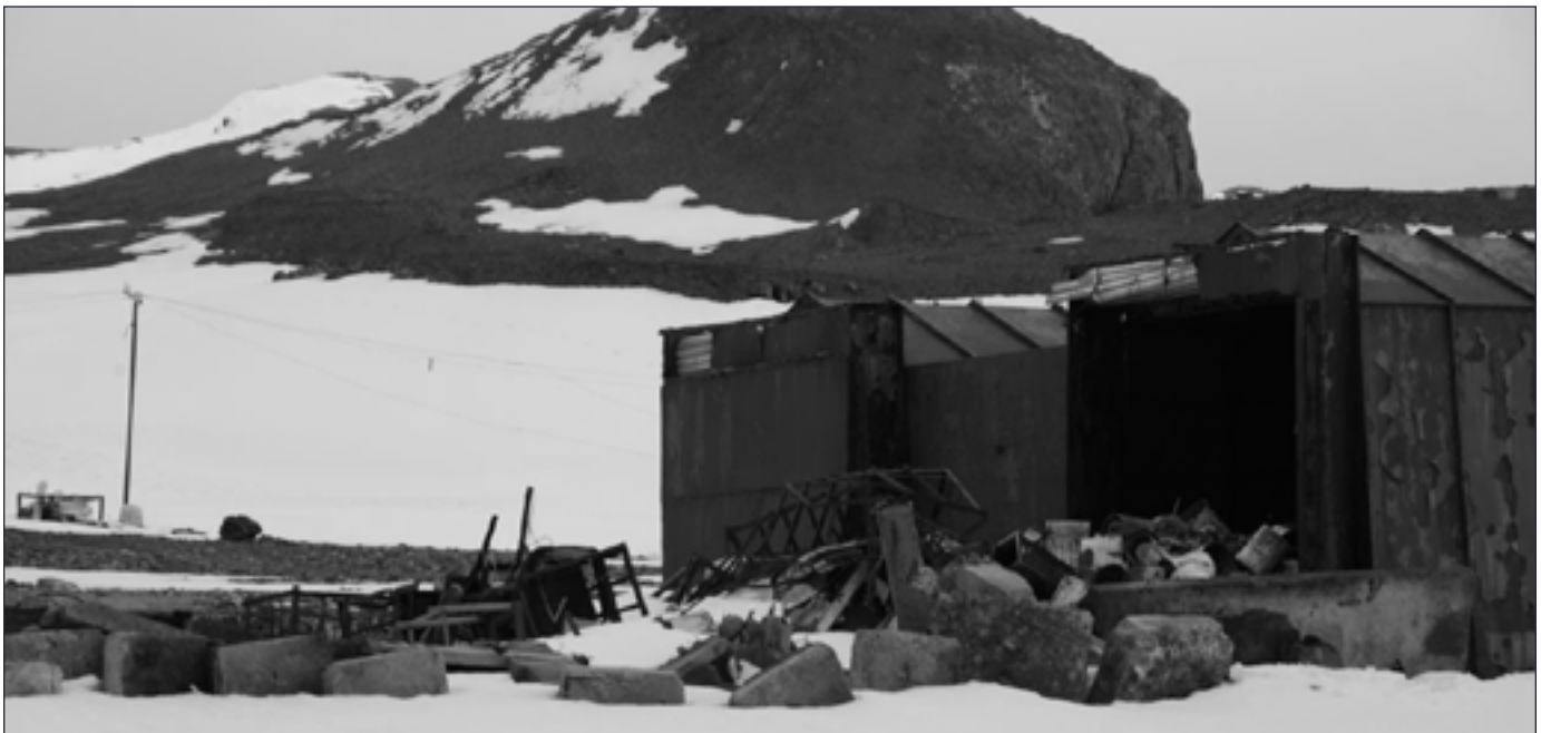
Great Wall Station, building
