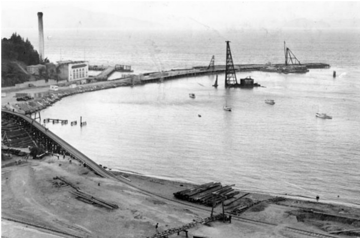
History #5. Municipal Pier under construction, and cove shoreline with State Belt Railroad tracks, 1932. (San Francisco Public Library Historic Photograph Collection, AAC 2288)
