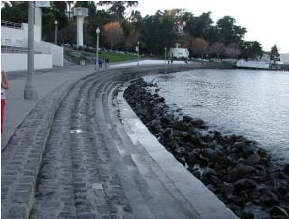
Buildings and Structures #6. Aquatic Park cove seawall, looking west, August 2000. (PGSO, CLI, SAFR, DSCN-2706)
