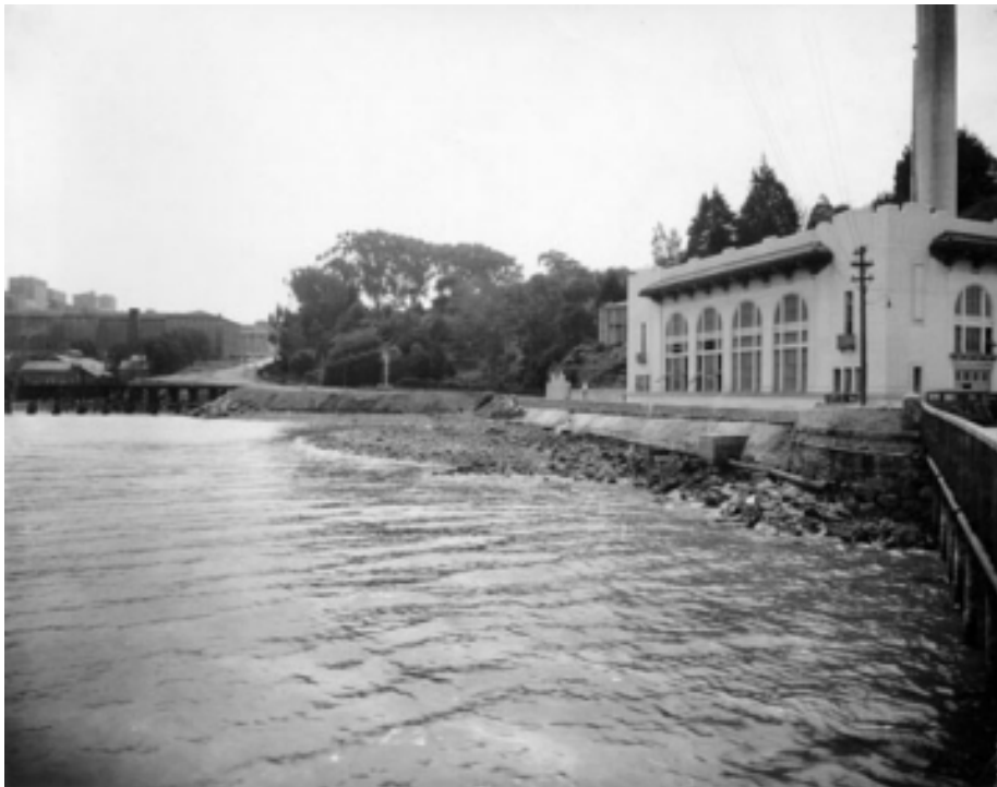
Vegetation #1. San Francisco Fire Department pumping station at foot of Van Ness, showing west boundary of Aquatic Park cove, looking south. (San Francisco Historic Photograph Collection, AAA 6726)
