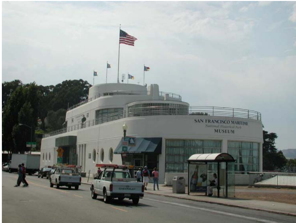
Buildings and Structures #1. Aquatic Park bathhouse, looking west along Beach St., August, 2000 (PGSO, CLI, SAFR, AP 0001)
