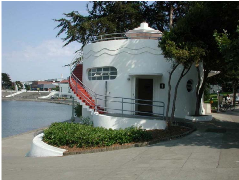
Buildings and Structures #2. West comfort station, looking southeast, August 2000. (PGSO, CLI, SAFR, DSCN-0002)
