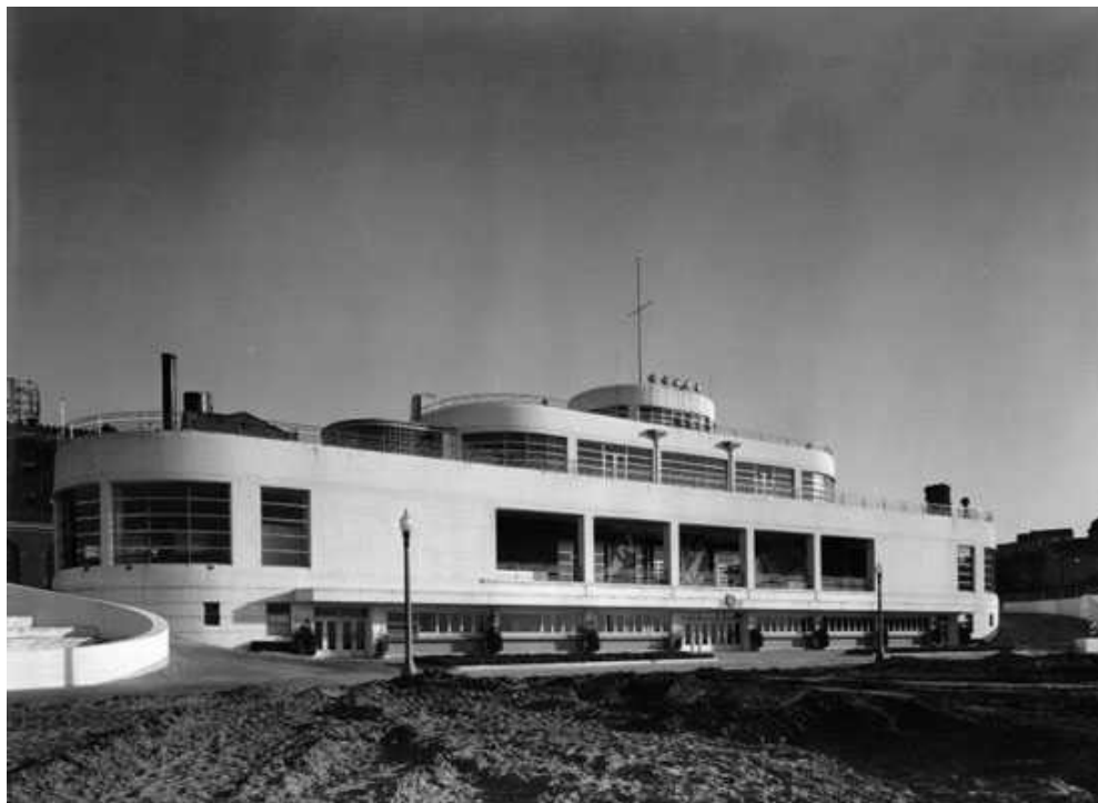
Vegetation #7. North elevation, Aquatic Park bathhouse, showing planting beds, n.d. (San Francisco Public Library Historic Photograph Collection, AAA 6748)
