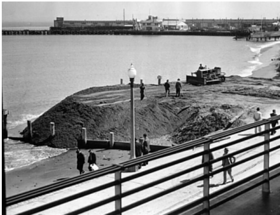
Topography #2. Sand moved from the Union Square parking lot excavation to fill in the beach, May 1941. (San Francisco Public Library Historic Photograph Collection, AAA 6699)
