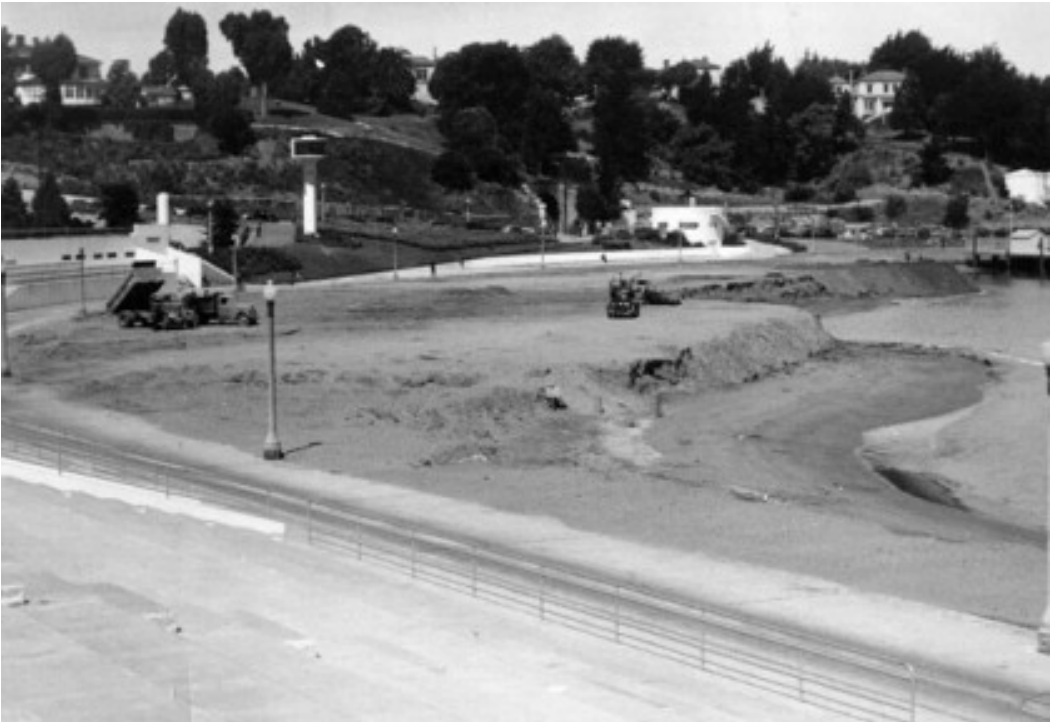
Topography #3. Spreading sand to create Aquatic Park beach, July 1941. (San Francisco Public Library Historic Photograph Collection, AAA 6701)
