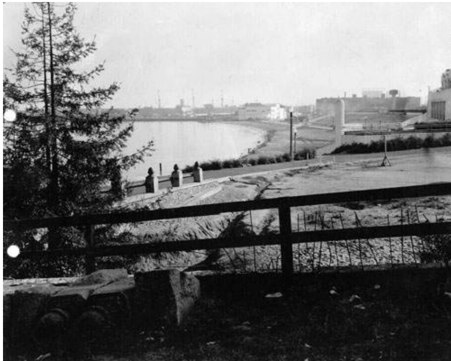
Small Scale Features #5. Wood post and rail fence atop Van Ness Avenue retaining wall provided a safety barrier between grade change, October 1942. (San Francisco Public Library Historic Photograph Collection, AAA 6717)
