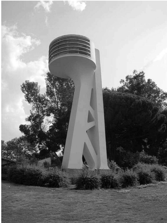
Buildings and Structures #7. West speaker tower, looking southeast, August 2000. (PGSO, CLI, SAFR, DSCN-0005)
