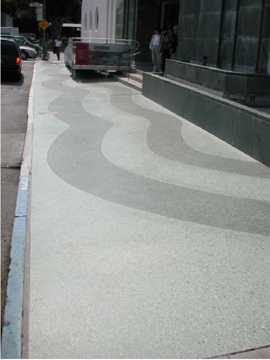
Circulation #6. Terrazzo wave pattern along Beach Street sidewalk in front of bathhouse, looking west, August 2000. (PGSO, CLI, SAFR DSCN-0077)
