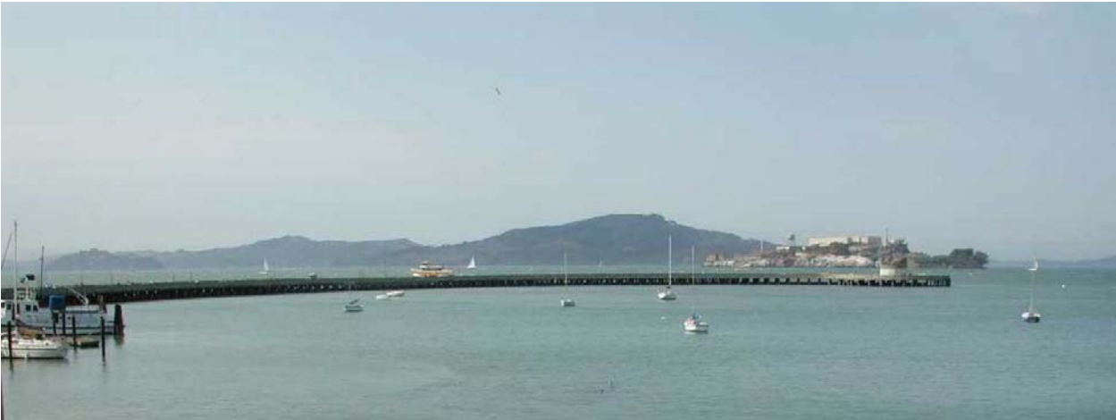
Circulation #2. Municipal Pier, looking north from the beach promenade, August 2000. (PGSO, CLI, SAFR, DSCN-0075)
