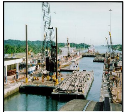
Previous method for conducting locks maintenance, with the lane fully closed to traffic for extended periods of time.
