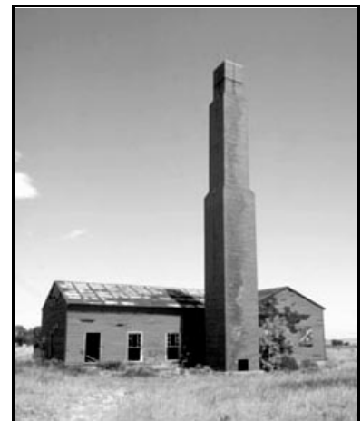
Hospital Boiler House Heart Mountain
