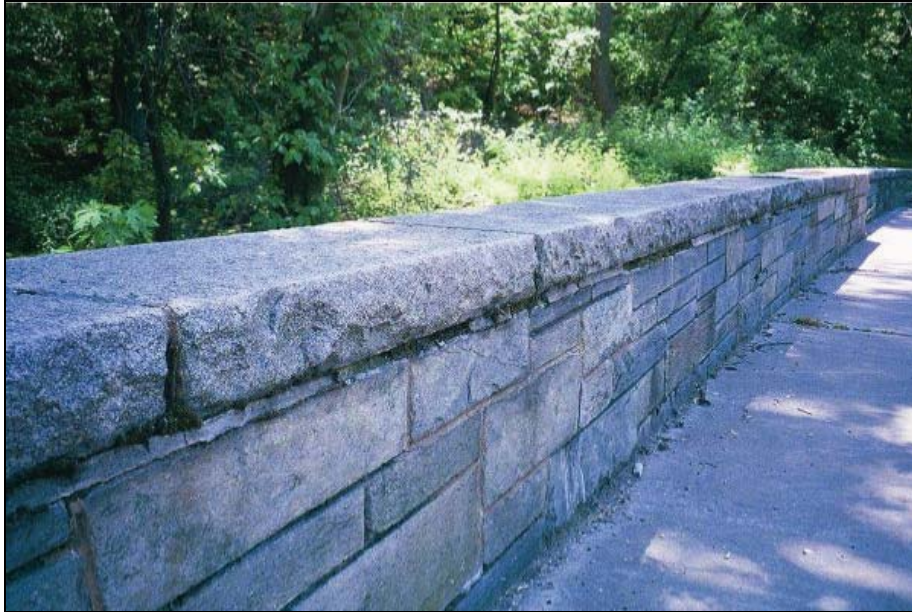
Figure B.10: Precast Concrete Guardwall Type 1, PCG
