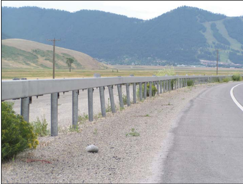
Figure B.4: Box Beam, G3
