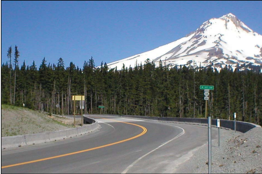
Figure B.7: Concrete Safety Shape, CSS
