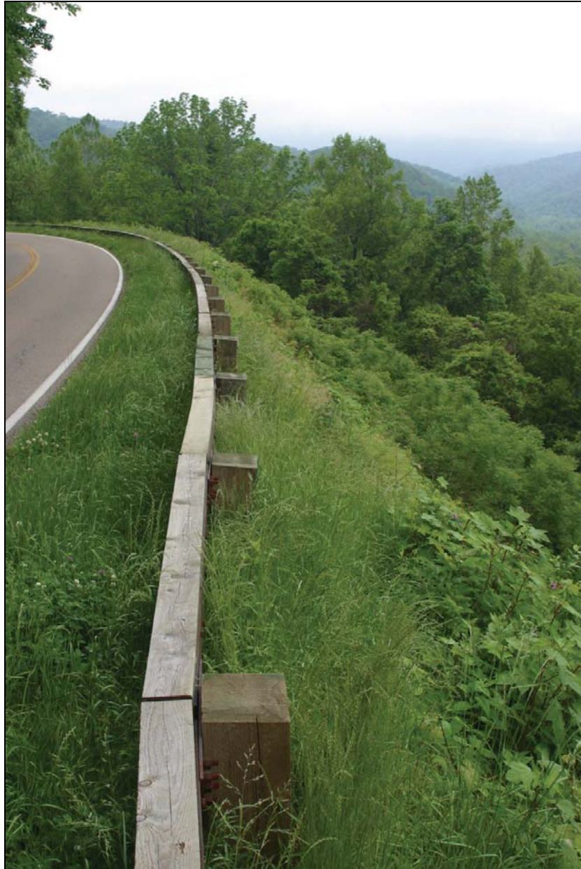
Figure B.9: Steel-Backed Timber Rail, SBT
