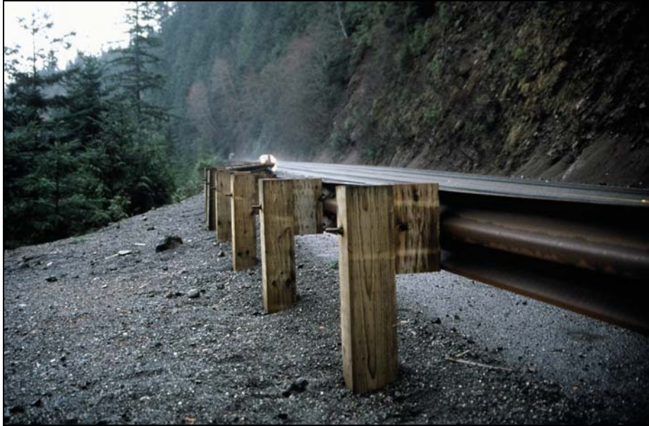
Figure B.5: Strong Post W-Beam, G4
