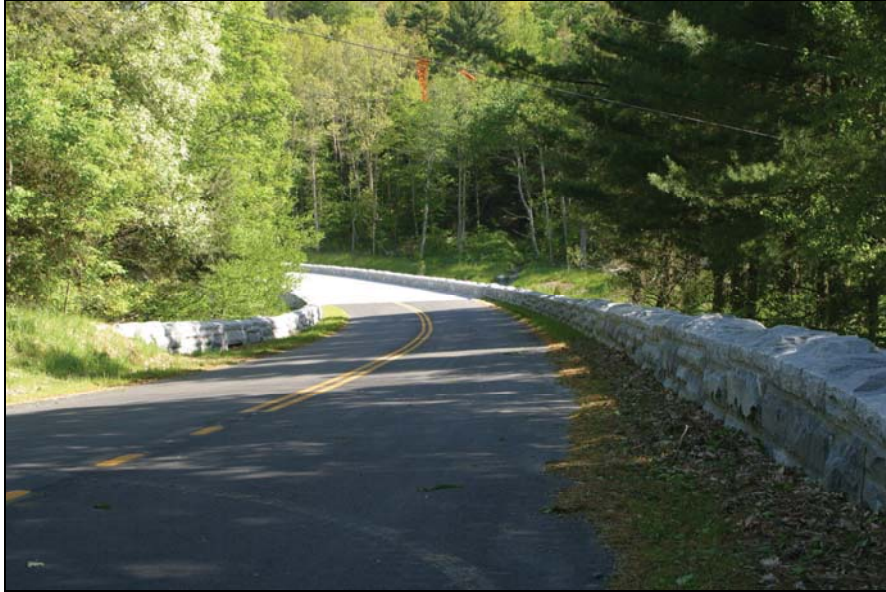
Figure B.11: Stone Masonry Guardwall, SMG
