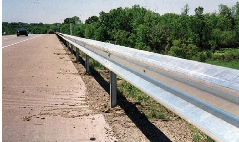
Figure B.3: Weak Post W-Beam, G2
