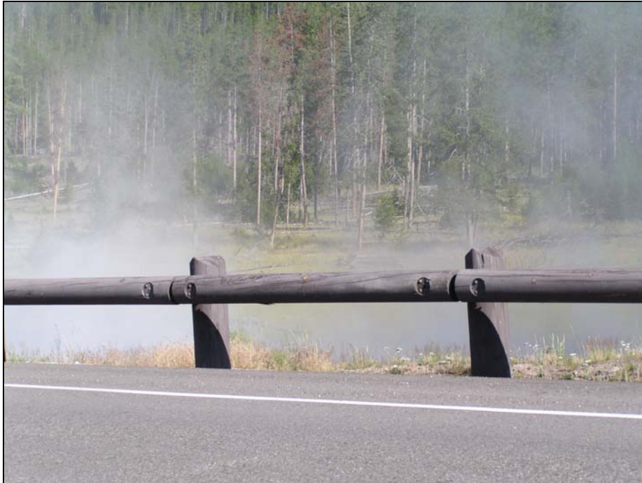
Figure B.8: Steel-Backed Log Rail, SBL
