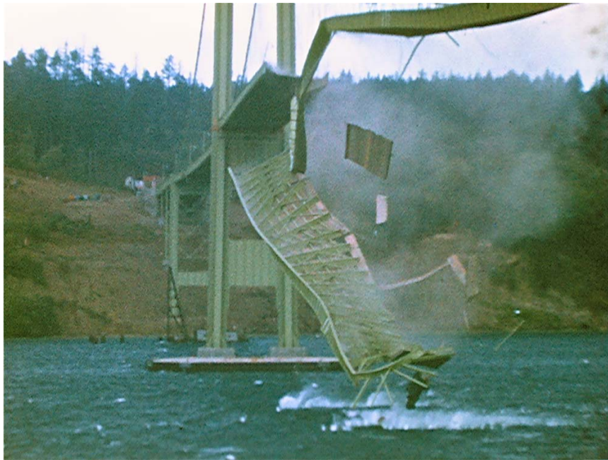
Figure 64. Collapse of Tacoma Narrows Bridge. (The Camera Shop, Tacoma WA)
