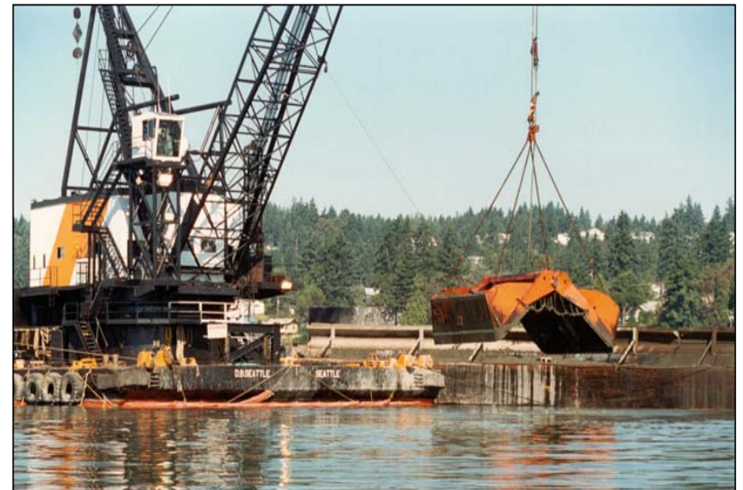
Remediating sediments at an MGP site
