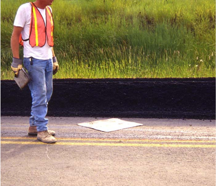
Exhibit 4-5 Obtaining Mixture Sample Prior to Compaction
