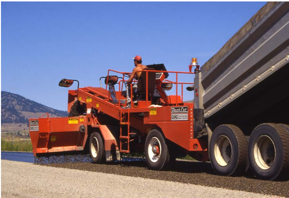
Exhibit 4-12 Chip Seal Aggregate Placement
