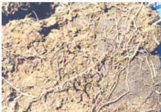
Figure C-9.0-1. Root intrusion into landfill cover soil
