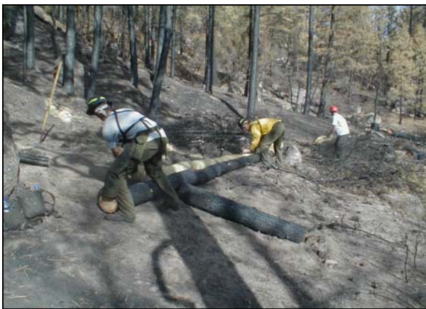
Log Erosion Barrier with Wattle
