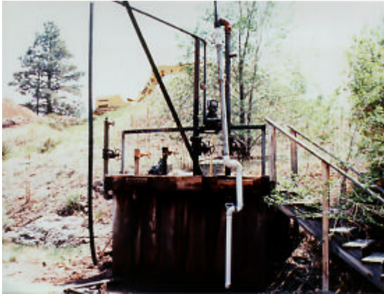
Former fill station
