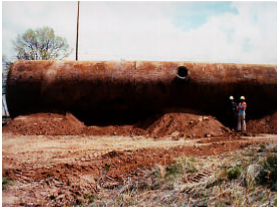
1988 Decommissioning activities ~ Tank 17
