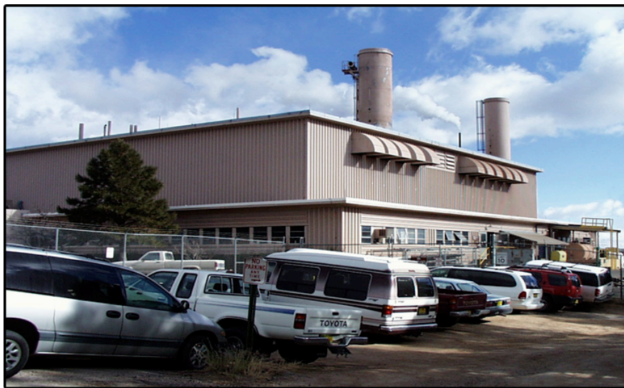
Figure 2.1-1 Main steam plant at TA-3 at LANL.
