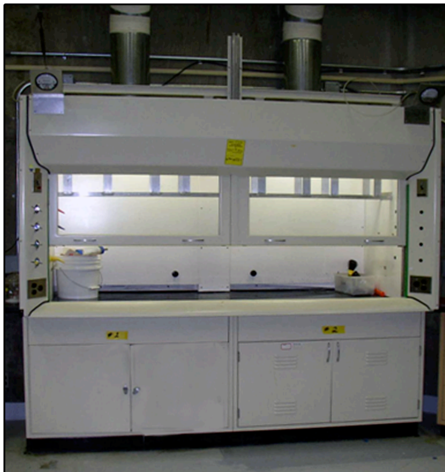
Figure 2.11-1 Example of a laboratory fume hood at LANL.
