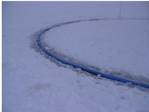
Picture 2: Completed skirt installation, February 2006
