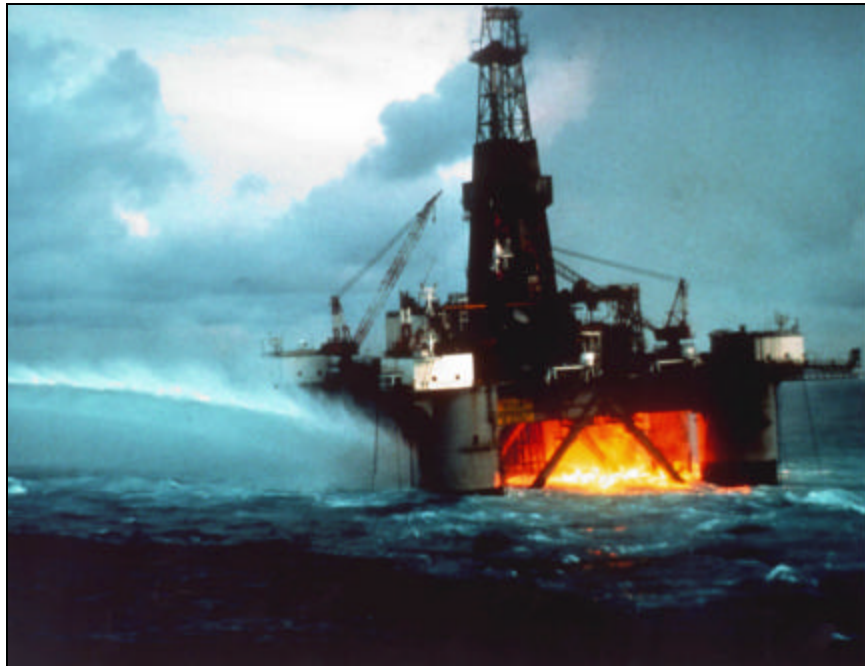
Figure 12 - Blowout and Fire from Failed Choke Line
