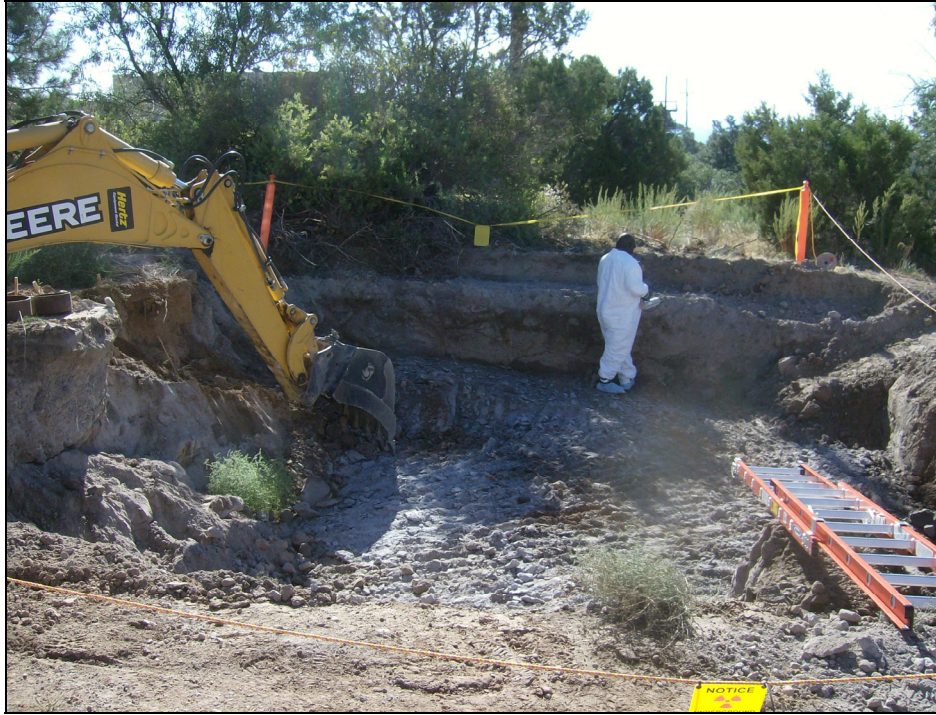
Photo 13 RCT surveying the boundary of excavated area, August–September 2007
