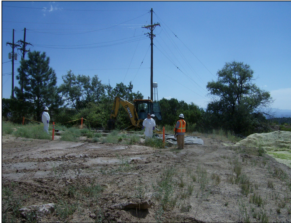
Photo 5 Preparation of area of elevated radioactivity for excavation, May 2007
