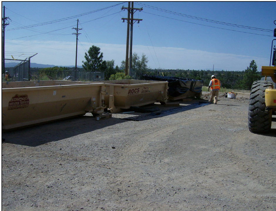
Photo 4 Mobilization of rolloff bins for excavated media, May 2007
