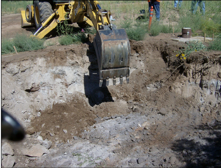
Photo 11 Excavation within northwest corner of area of elevated radioactivity, August–September 2007
