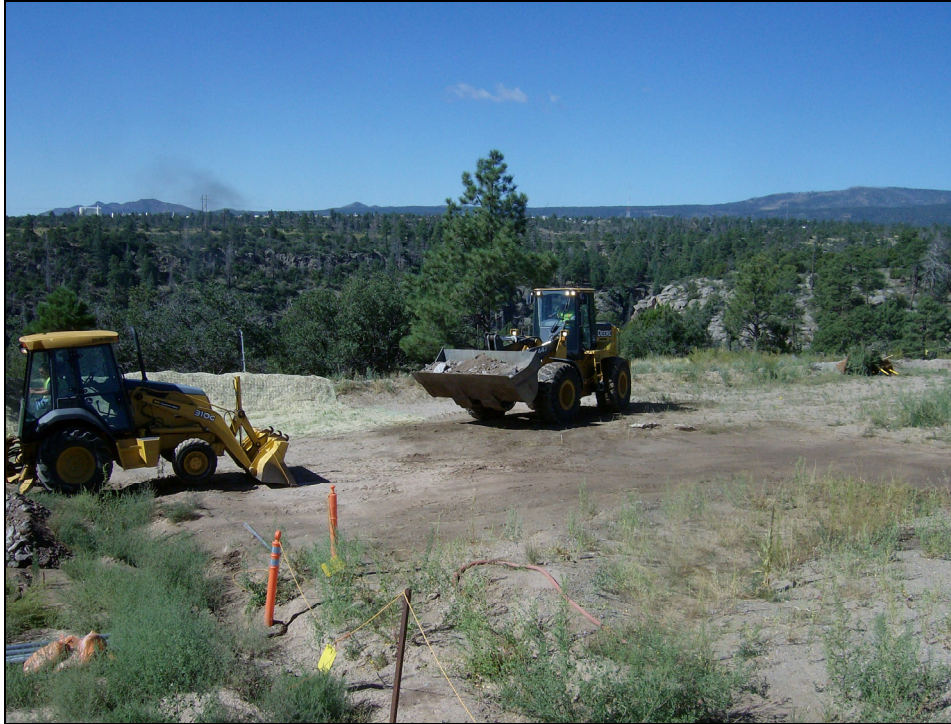
Photo 9 Front-end loader transport of removed soil to rolloff bins, August–September 2007
