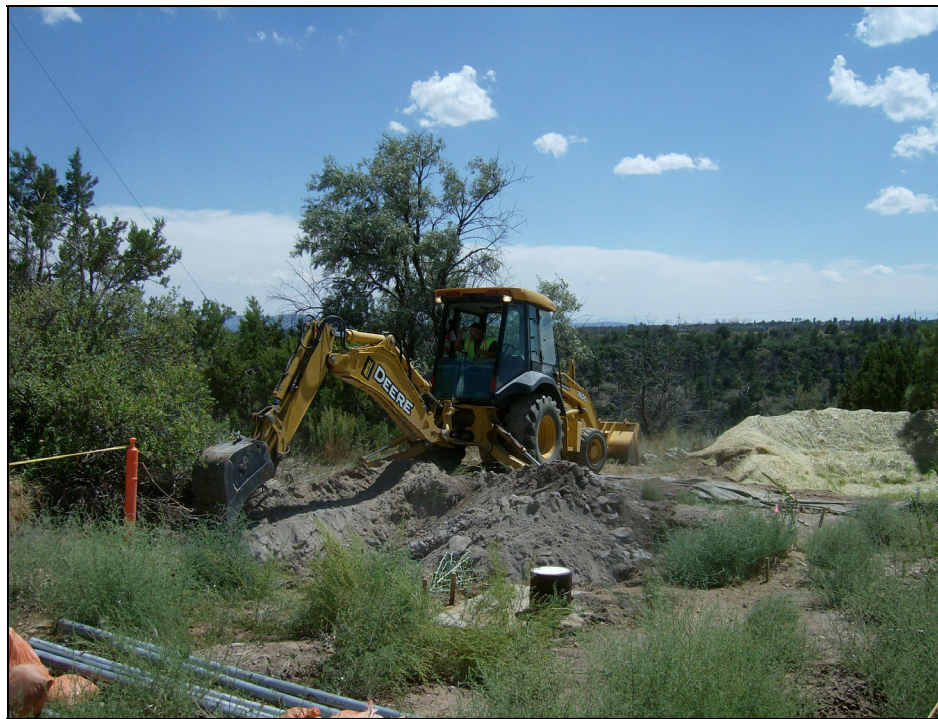
Photo 6 Excavation of area of elevated radioactivity, August–September 2007
