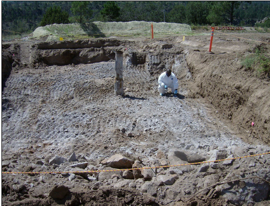
Photo 15 Area of excavation (view to the south), September 2007
