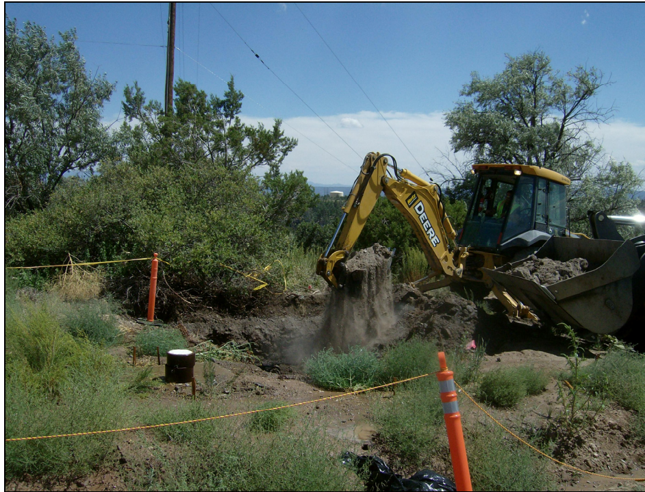
Photo 7 Excavation of elevated area of radioactivity, August-September 2007
