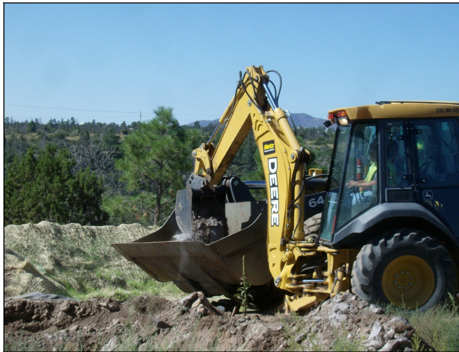
Photo 8 Transfer of removed soil to front-end loader, August-September 2007
