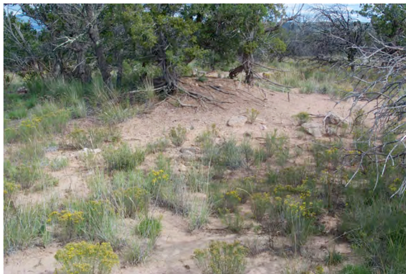
Figure 13. Trail Segment 2C and SWEIS 130, a one- to three-room room structure, impacted by severe erosion.
