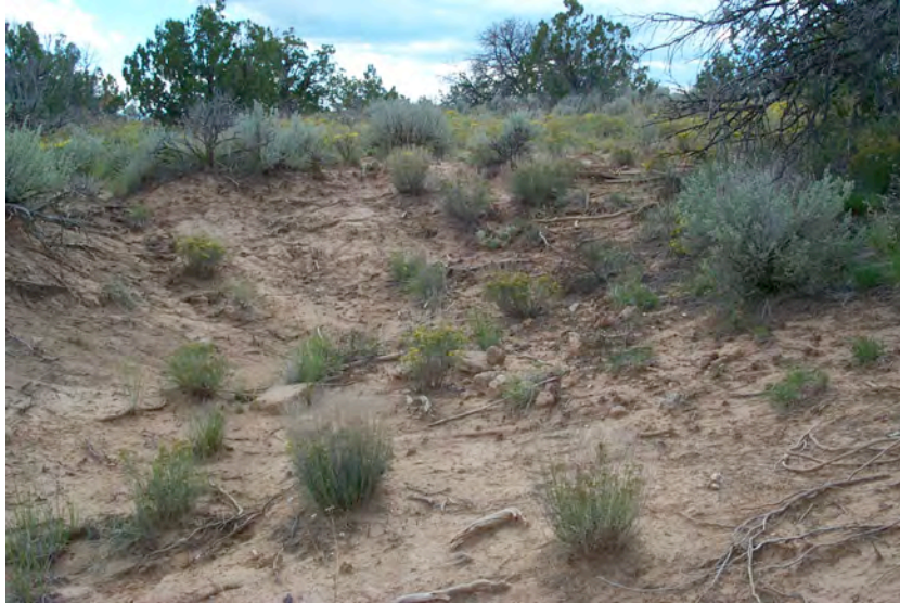
Figure 12. Trail Segment 2C and SWEIS 129, a one- to three-room structure, impacted by severe erosion.
