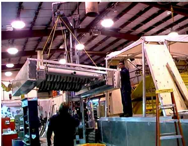
Lifting recovery unit on board work platform.
