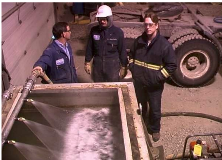
Chosen nozzles installed on spraybar.
