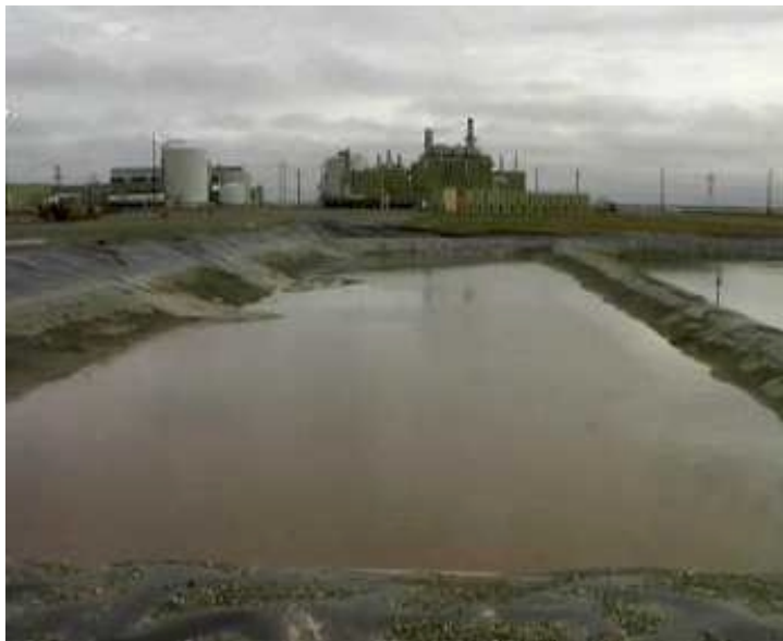
Test pit with Saltwater Injection Plant (SIP) in background.
