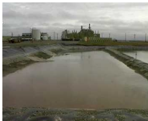
Figure 2.5 Test pit with Saltwater Injection Plant in the background.
