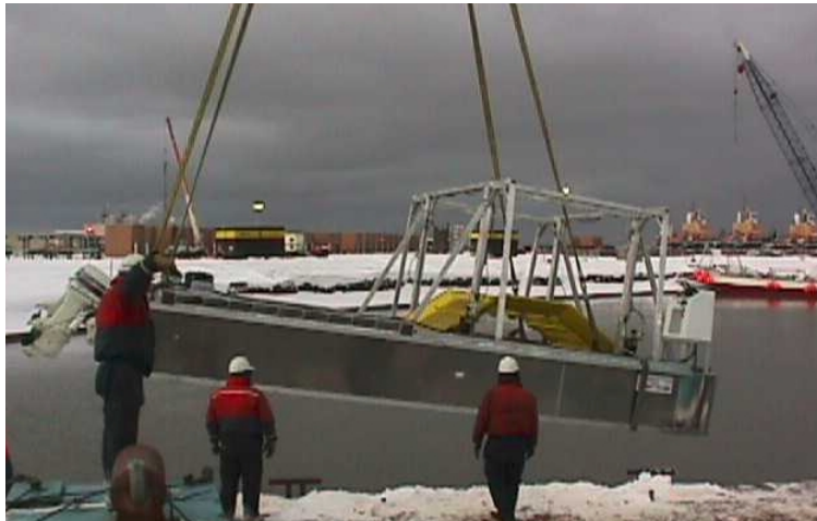
Work platform lifted for deployment.
