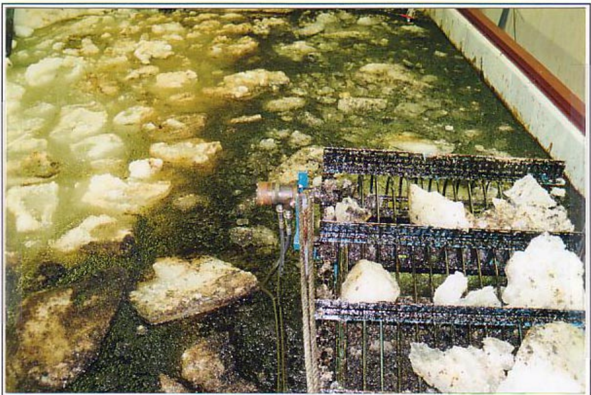
The Lifting Grated belt operating in conditions with much slush and ice pieces up to 50 cm . Ice on the belt has been cleaned with a water flushing system.
