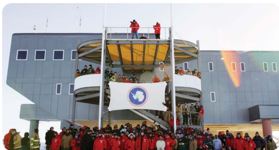
In January 2008, honored guests joined with NSF to dedicate the Amundsen-Scott South Pole Station. The new, elevated station is larger and much more sophisticated than any previous structure built at the Pole—a reflection of the logistical support needed for the ever-increasing range and diversity of the research taking place there. Credit: Peter Rejcek, National Science Foundation
