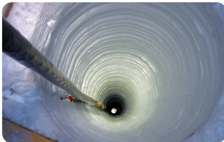
A view of the signal cables from strings of Digital Optical Modules (DOMs) extending down into the ice. The IceCube Neutrino Observatory, under construction in the highly transparent ice beneath the surface of the South Pole, will be composed of 70 strings of DOMs and 140 surface cosmic ray air detector modules. Credit: Kathie L. Olsen, National Science Foundation
