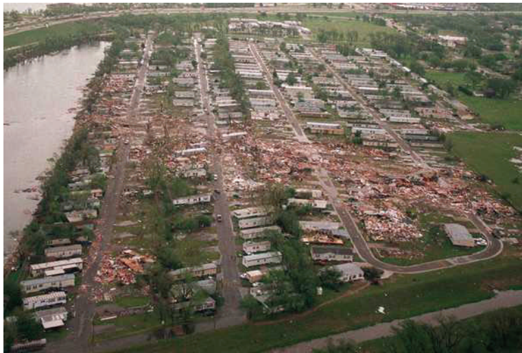
An aerial view of the damage at Lakeshore Mobile Homes Resort. Picture by Travis Heying/The Wichita Eagle
