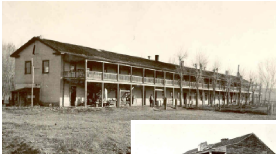
Old Fort Laramie Cavalry Barracks, 1909 Construction Photograph Albums, 1903-66 Office of the Chief Engineer RG 115, Records of the Bureau of Reclamation NARA-Rocky Mountain Region, Denver
